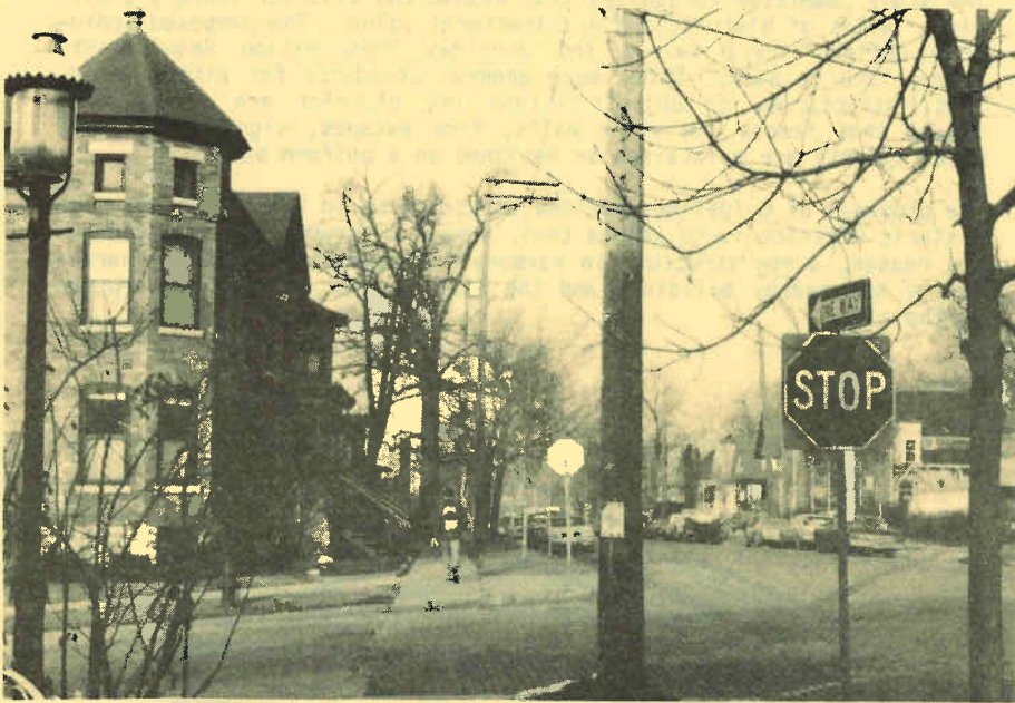
Looking northeast from the corner of Detroit and East Kingsley Streets.
