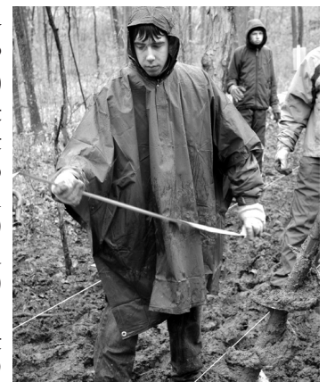
Allen Eyler installing a boardwalk at Brown Park
