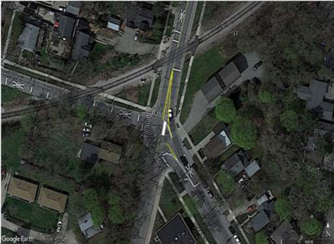
Short Term - Add pavement markings to better delineate vehicle paths through intersection.
