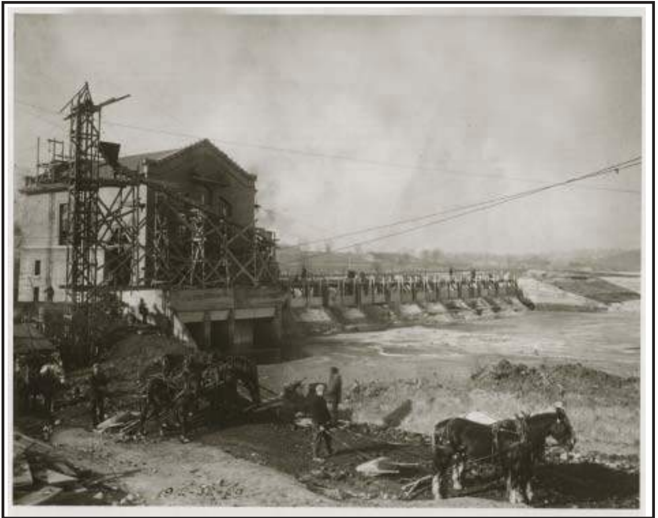
Construction of Barton Dam - 1927
