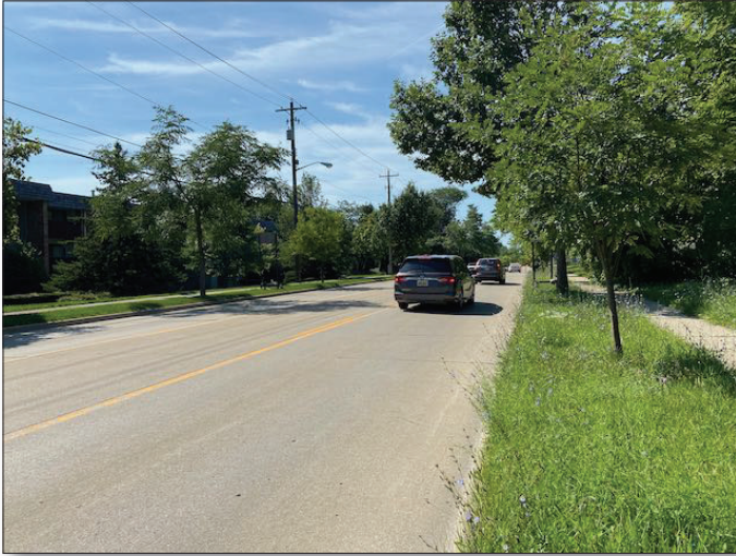
View South of South Maple Road
