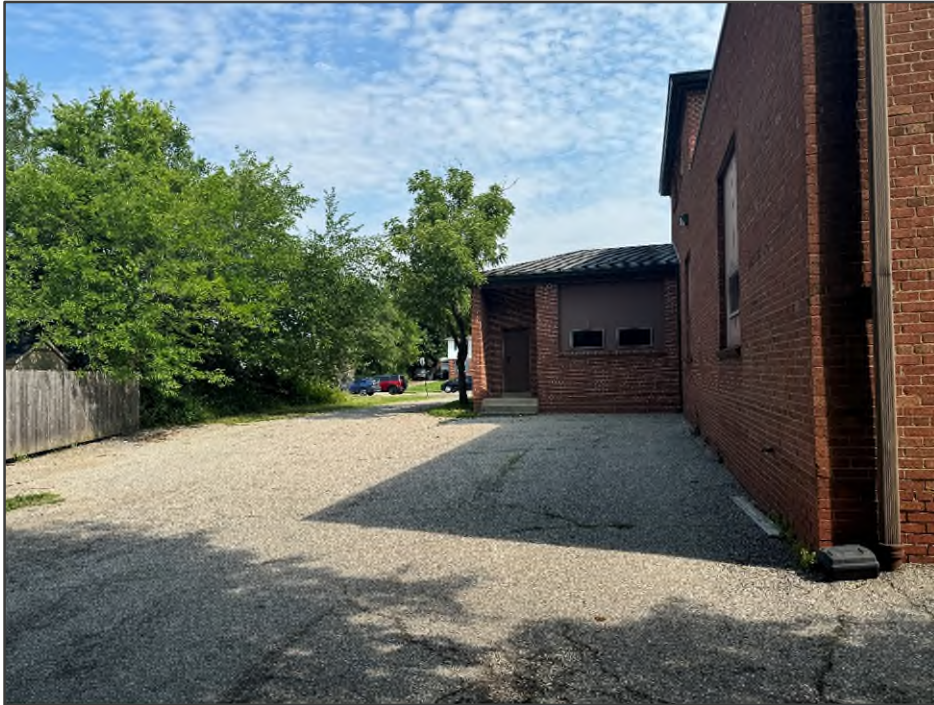
PHOTO NO. 15: View of the western parking lot area.
