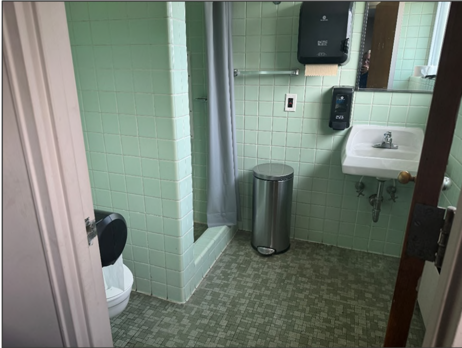
PHOTO NO. 21: View of a second-floor restroom.
