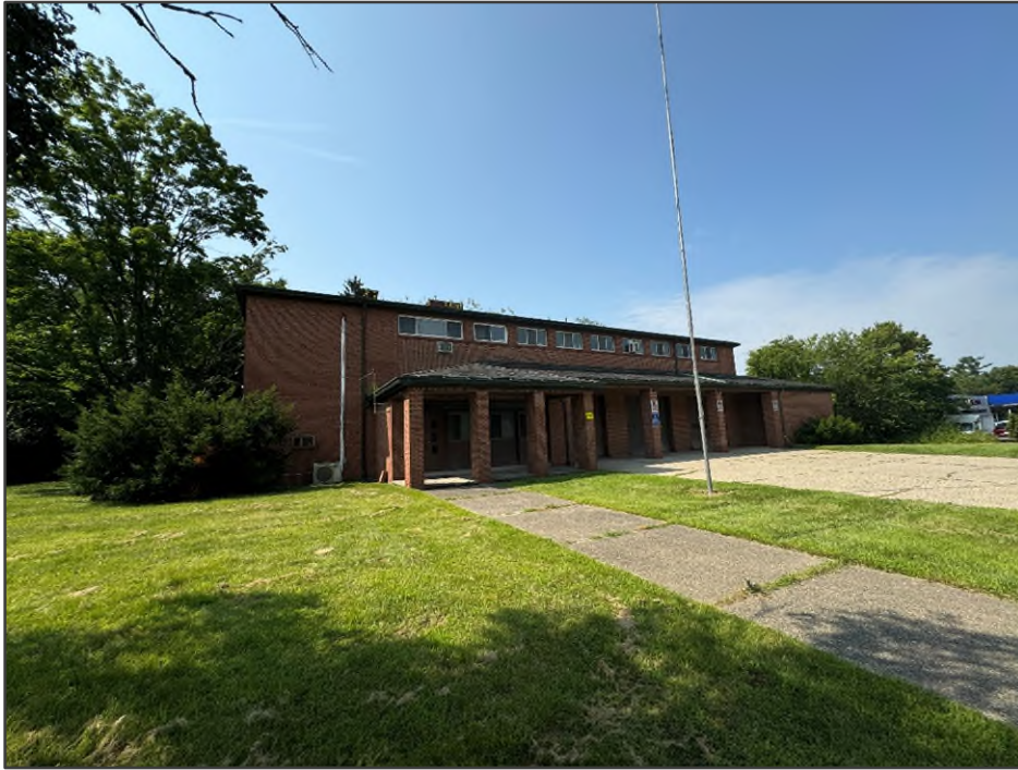
PHOTO NO. 1: View of the former fire station building, 1510 East Stadium Boulevard.
