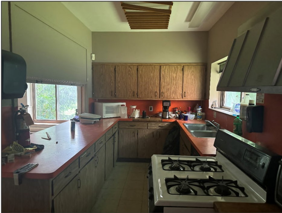
PHOTO NO. 16: View of the first-floor kitchen area.
