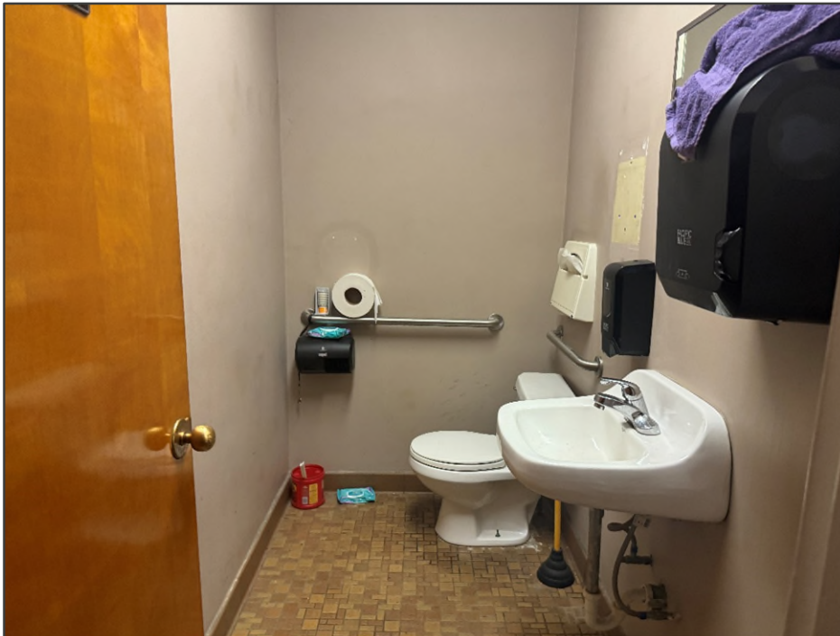
PHOTO NO. 18: View of a first-floor restroom.
