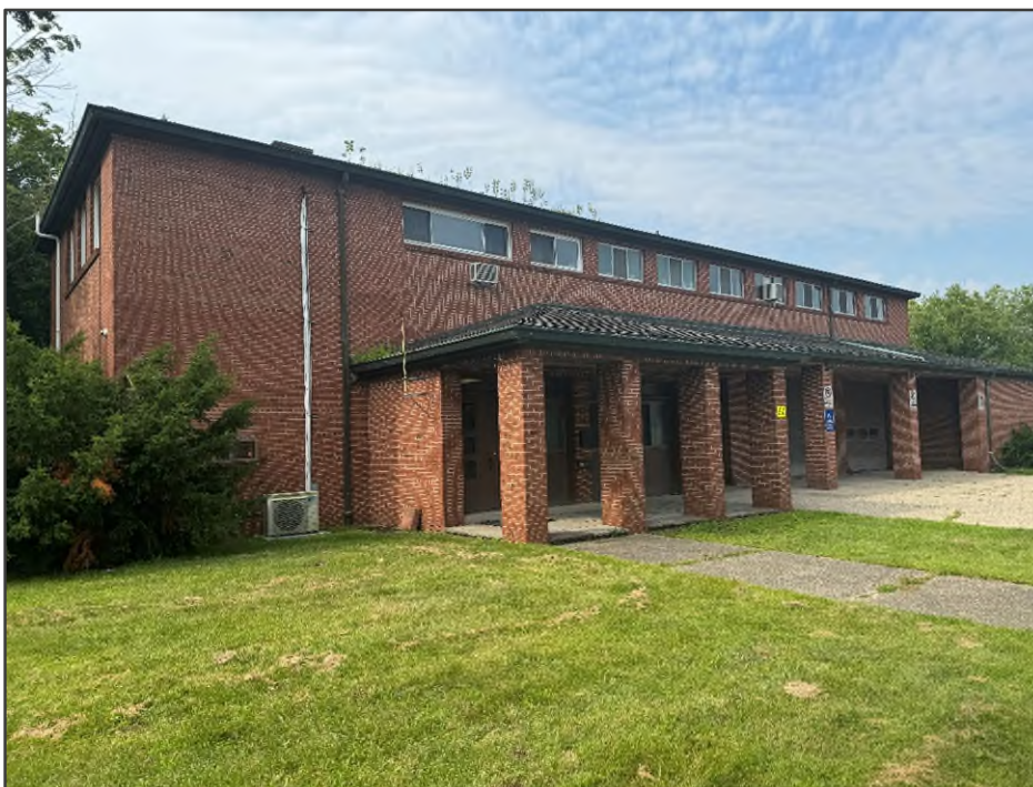
PHOTO NO. 8: View of the front garage bay portion of the building.
