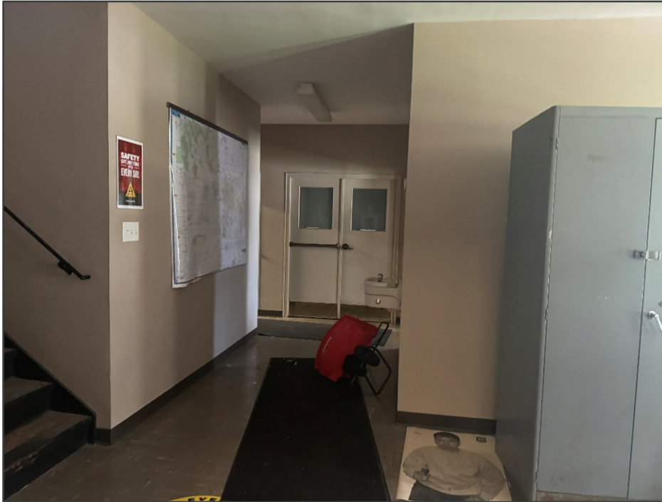
PHOTO NO. 17: View of a central first floor hallway.
