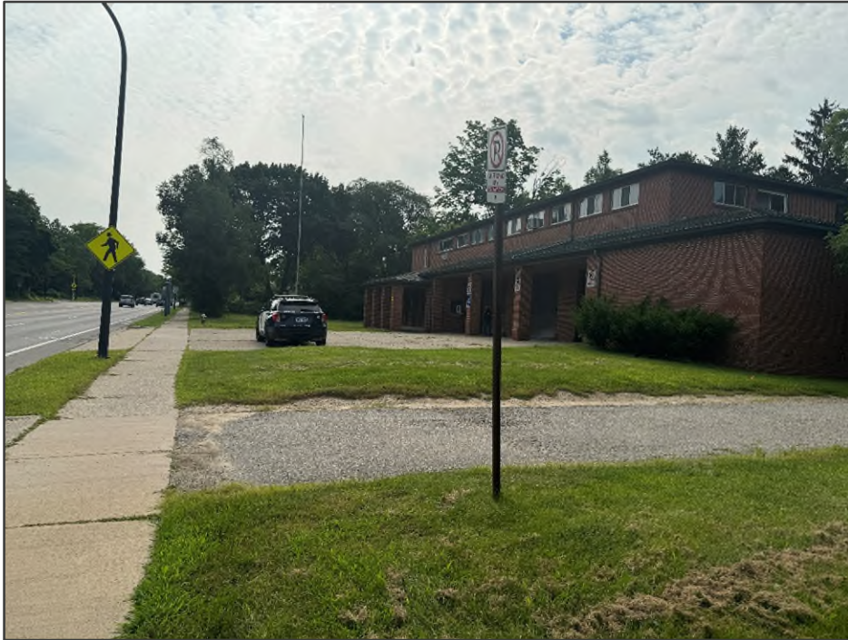
PHOTO NO. 3: View of the northern Subject Property boundary
