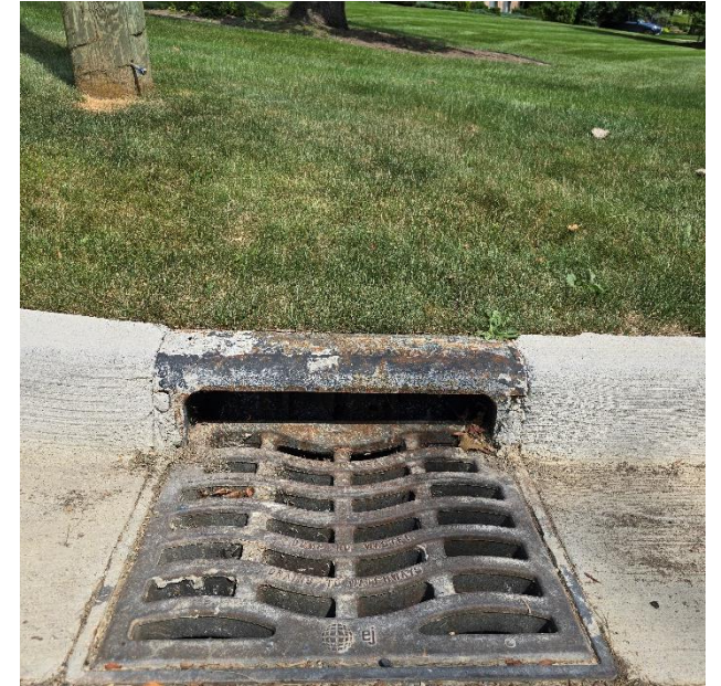
Improved roadway drainage
