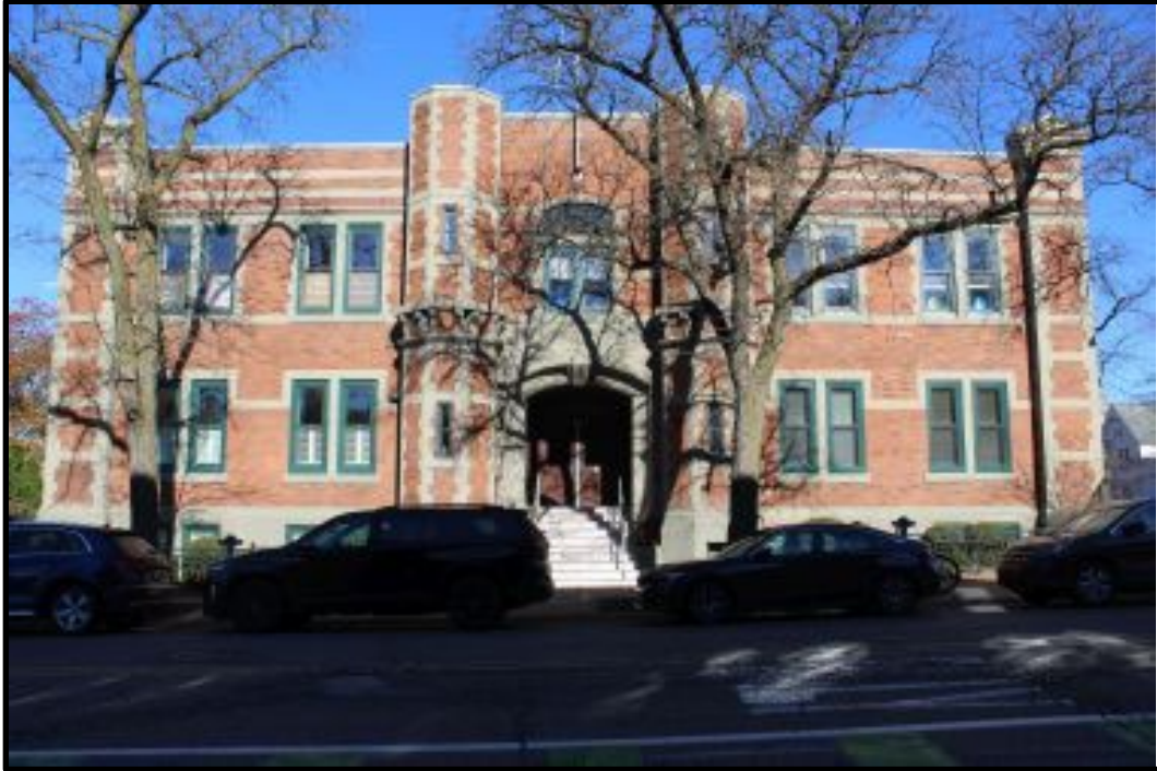
Figure 5-29. Ann Arbor Armory, 233 East Ann Street, view from the North .
