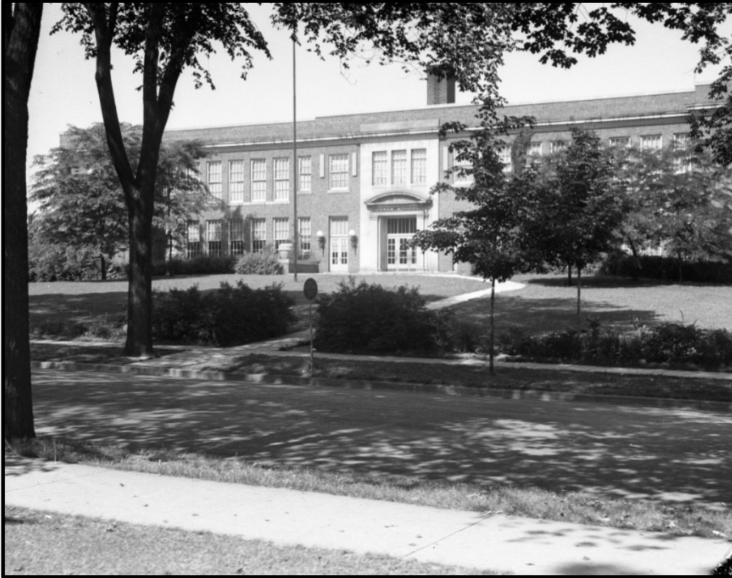
Figure 5-12. Community High School, 401 North Division Street, view to the North west, 1935.
