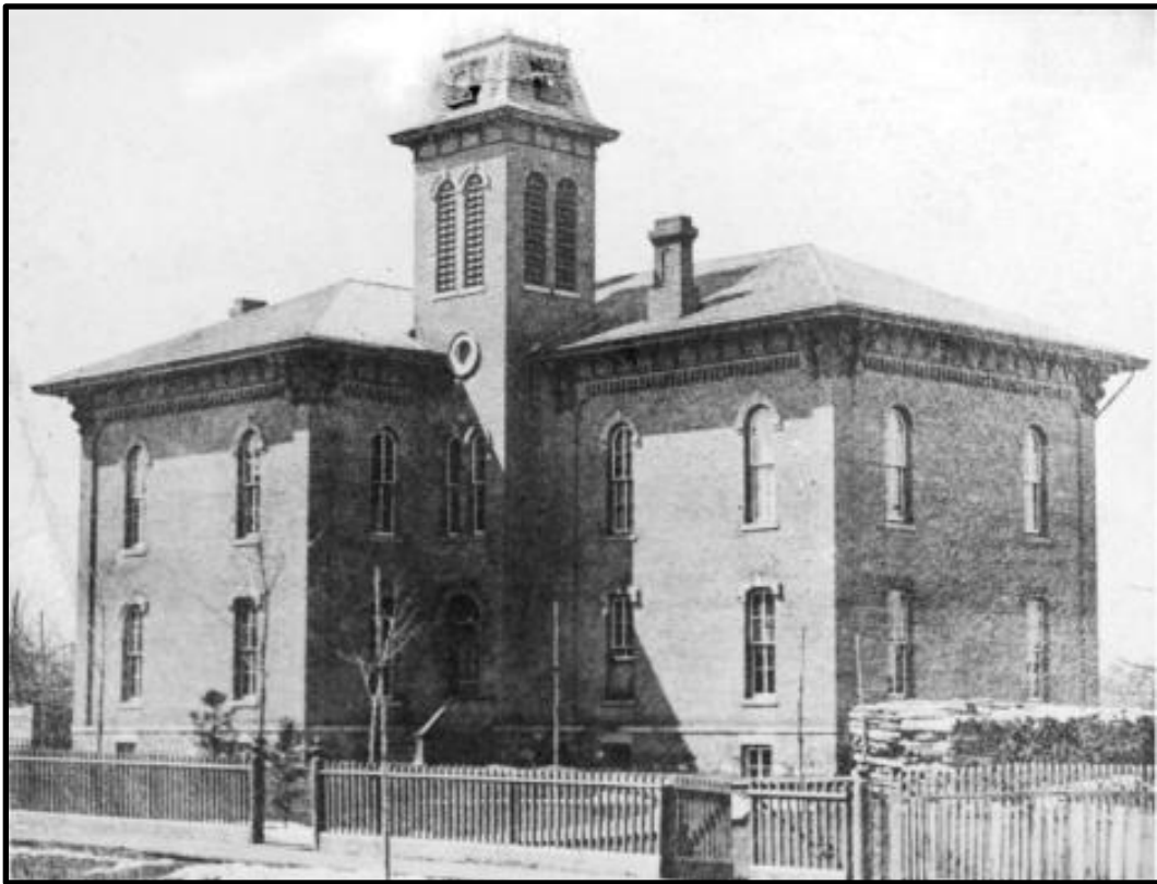
Figure 5-11. Undated photograph showing the 1867 Fourth Ward School.
