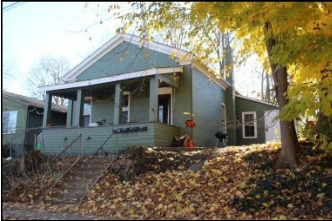
Figure 5-23. Former Union Church at 504 High Street, view to the southeast.
