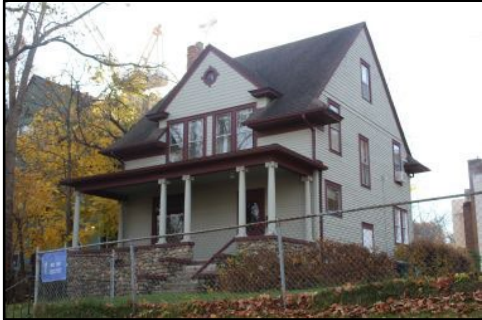
Figure 5-26. University Reformed Church/Harvest Mission Community Church Rectory at 1001 East Huron Street, view from the southeast.
