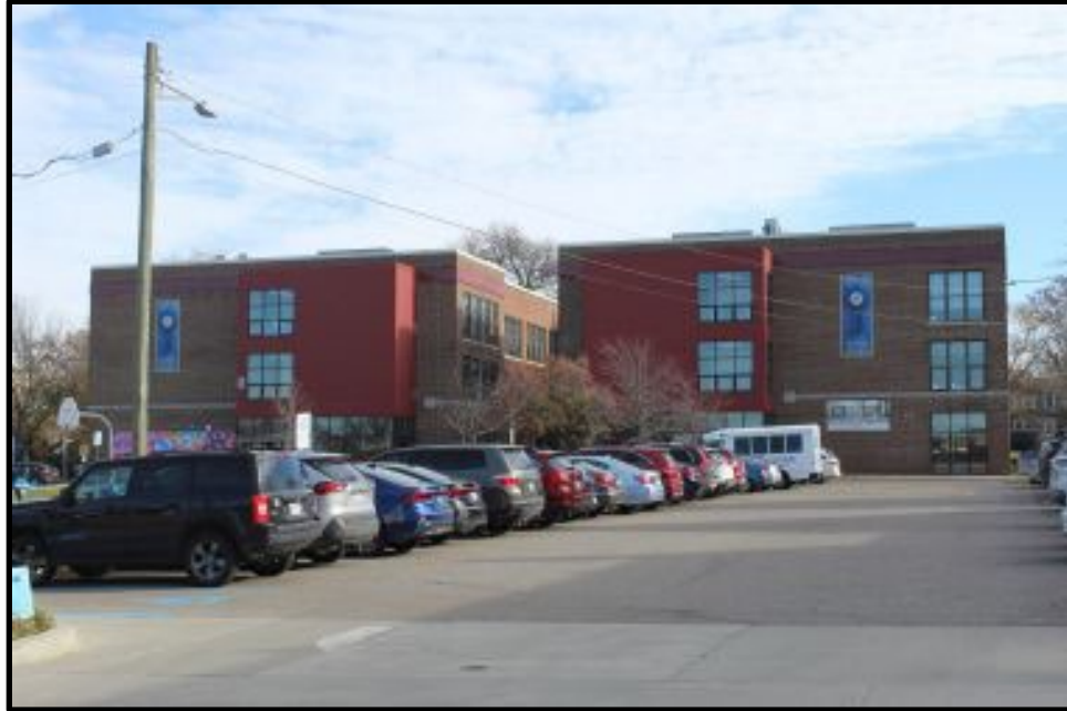
Figure 5-14. Community High School, 401 North Division, view to the south 2023.
