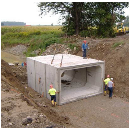
Figure 32: Example of a box culvert
