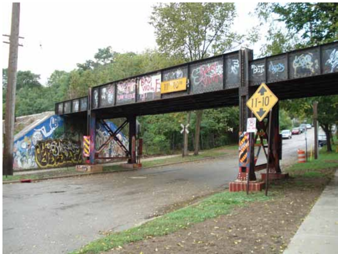
Figure 25: Northern segment of the railway elevated.
