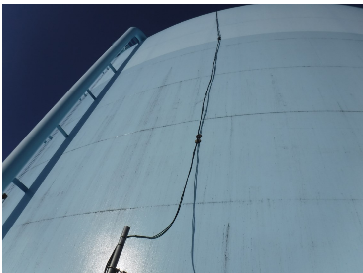
15) Antenna cables are attached with magnets on the sidewall.
