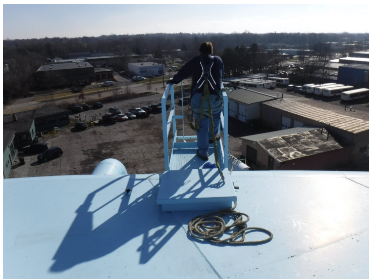
18) Step-off platform and hatch on the roof.
