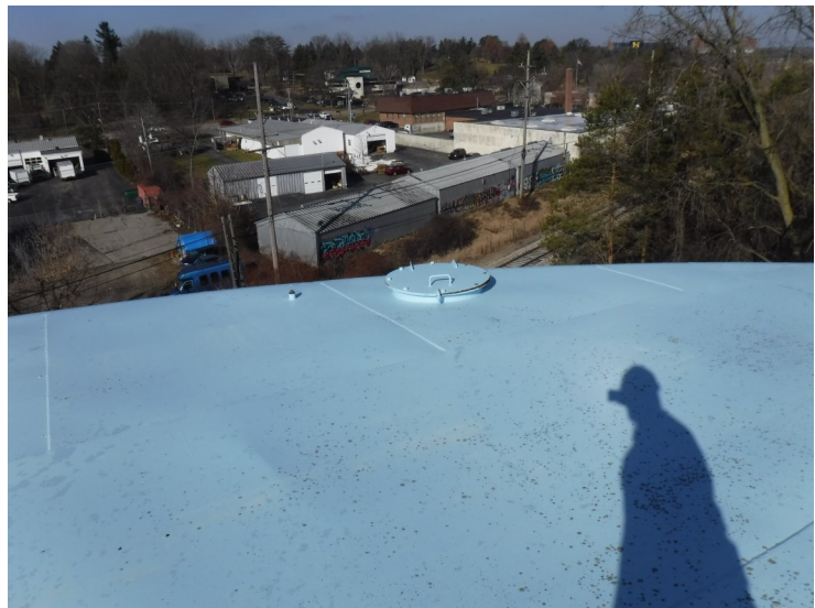
26) Bolted ventilation hatch on the edge of the roof.
