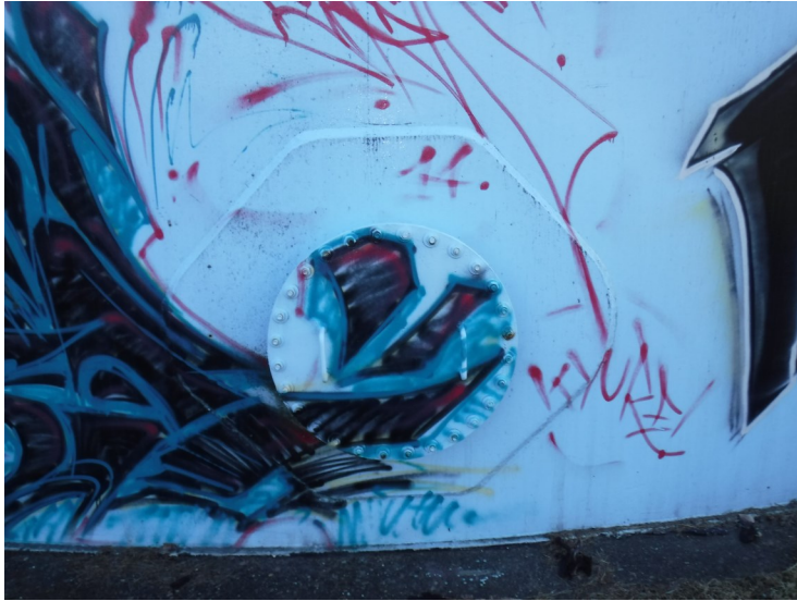
13) Second sidewall manway.
