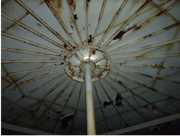
37) Center of the roof with ring stiffener and column.
