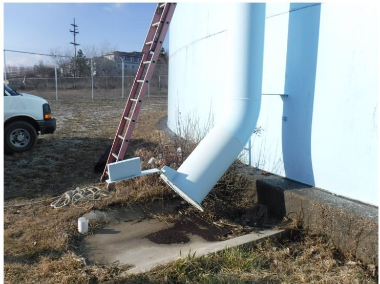
11) The overflow pipe discharges to a concrete splash pad and has a flap gate that is in good condition.
