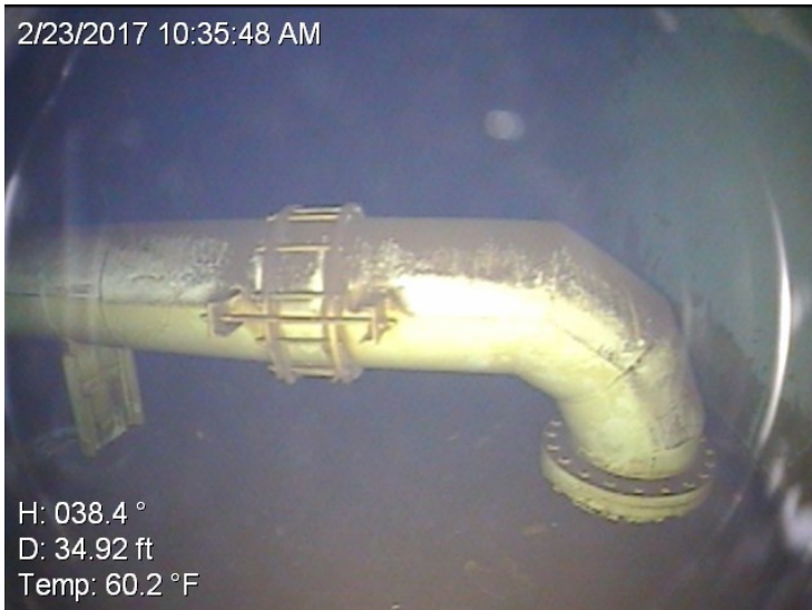
52) Fill pipe penetration through the floor.
