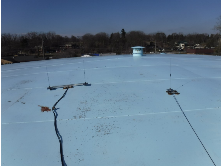
25) Antennas attached to the roof with magnets.
