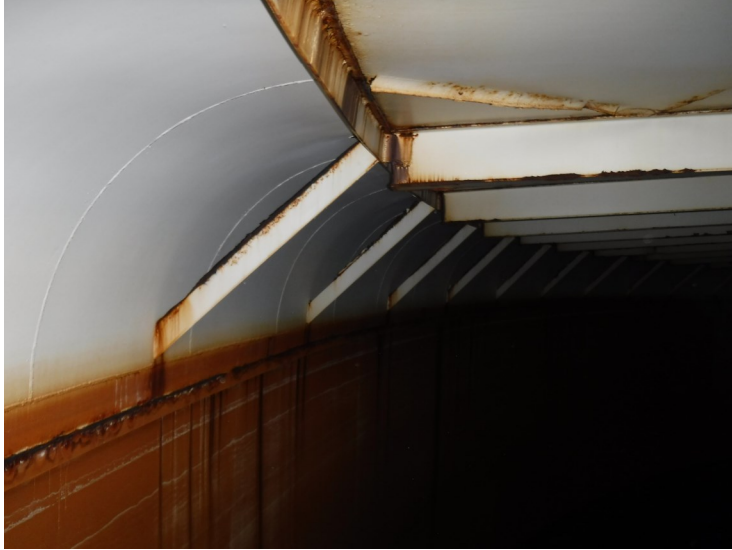
28) Wet interior roof knuckle wind girder and kickers at the stiffeners.
