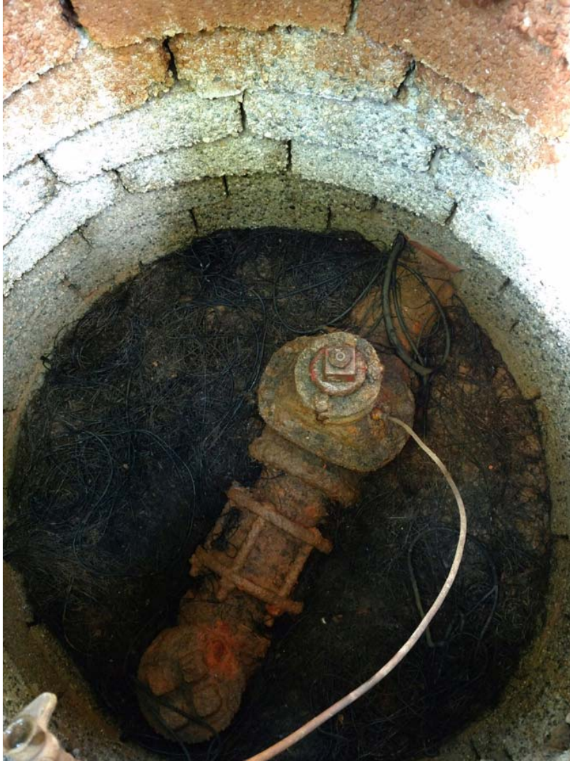
Well 5E Shutoff Valve
