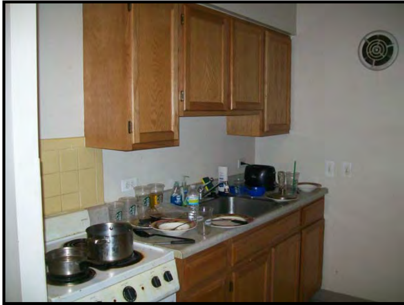
PHOTOGRAPH NO. 13: SUBJECT BUILDING: TYPICAL VIEW OF TENANT UNIT KITCHEN
