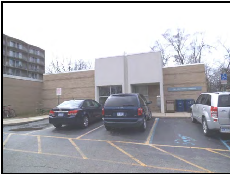
PHOTOGRAPH NO. 2: OFFICE PORTION OF SUBJECT BUILDING AS VIEWED FACING WEST
