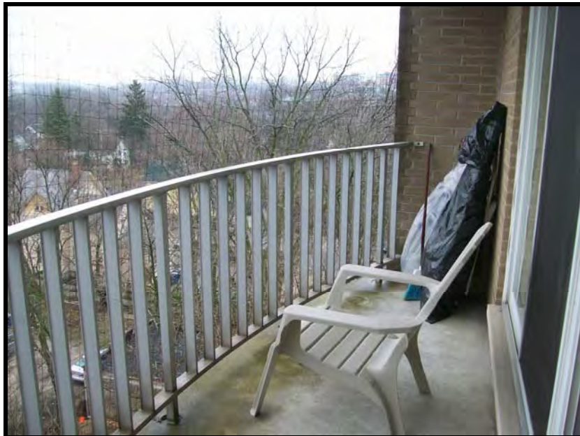
PHOTOGRAPH NO. 12: SUBJECT BUILDING: TYPICAL VIEW OF TENANT UNIT BALCONY
