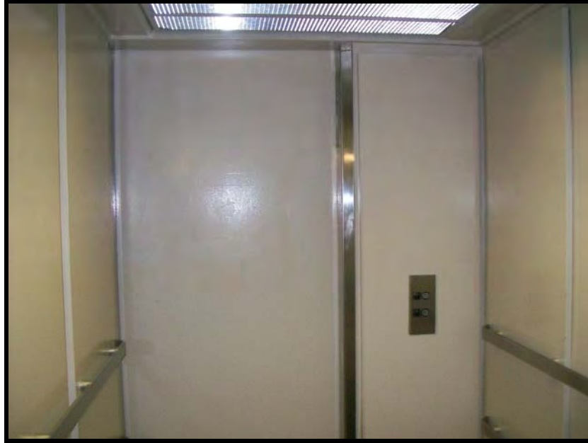
PHOTOGRAPH NO. 19: SUBJECT BUILDING: VIEW OF ELEVATOR INTERIOR
