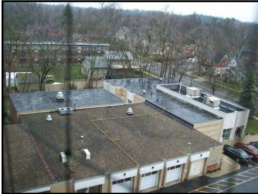
PHOTOGRAPH NO. 22: SUBJECT BUILDING: VIEW OF ROOF OVER OFFICE WING
