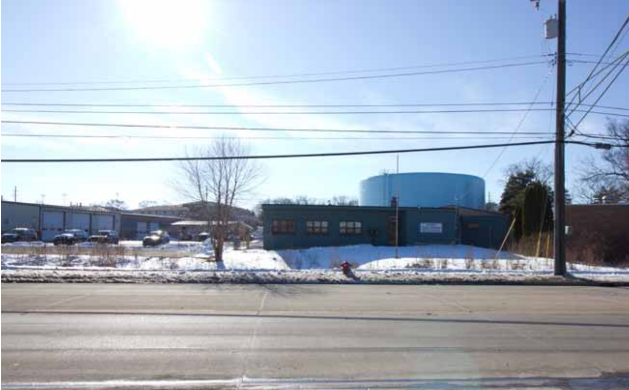
View of existing buildings
