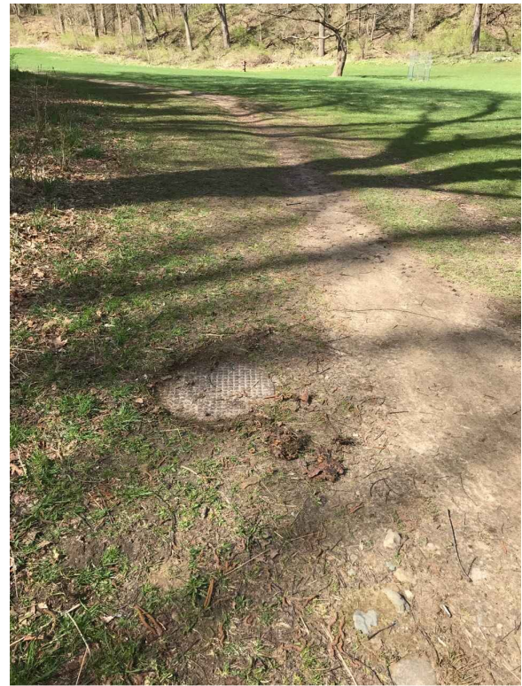
71-70030 RIM: 794.90 INVERT ELE: 789.90 PHOTO LOOKING WEST
