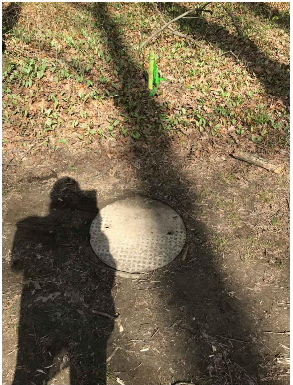
71-70044 RIM: 787.14 INVERT ELE: 781.14 PHOTO LOOKING SOUTHWEST
