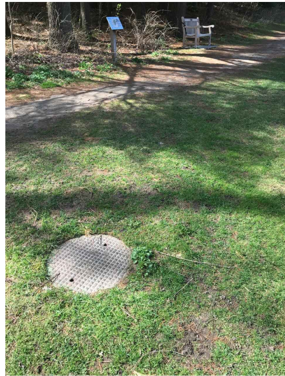
71-70032 MH SLIGHTLY OFFSET. RIM: 816.76 INVERT ELE: 811.65 PHOTO LOOKING WEST
