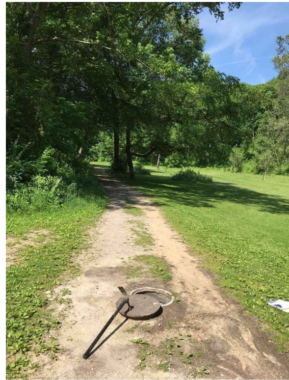
71-70043 RIM: 788.60 INVERT ELE: 783.00 PHOTO LOOKING WEST
