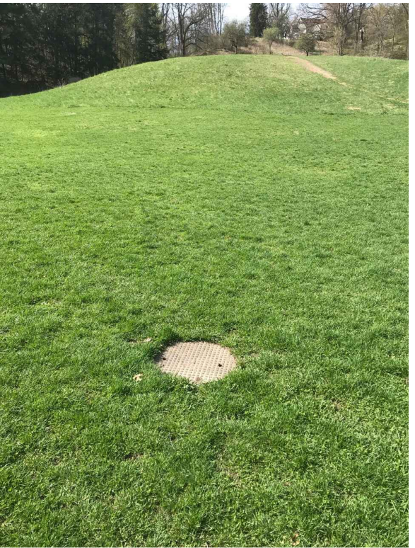
71-70031 RIM: 807.70 INVERT ELE: 802.75 PHOTO LOOKING SOUTH
