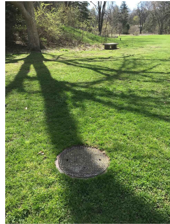
71-70029 RIM: 801.21 INVERT ELE: 797.08 PHOTO LOOKING WEST
