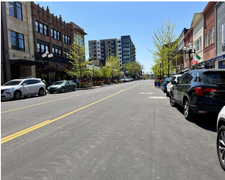
Main Street Resurfacing Project
