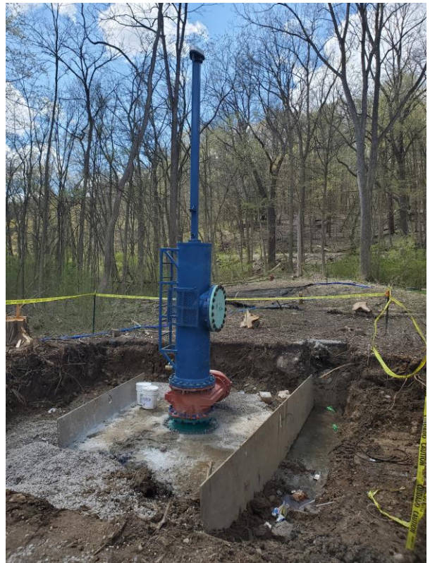
Barton Pump Station Valve Replacement Project
