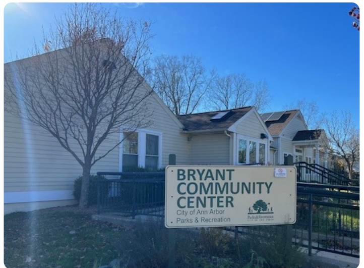
The Bryant Community Center, where geothermal drilling began recently.
