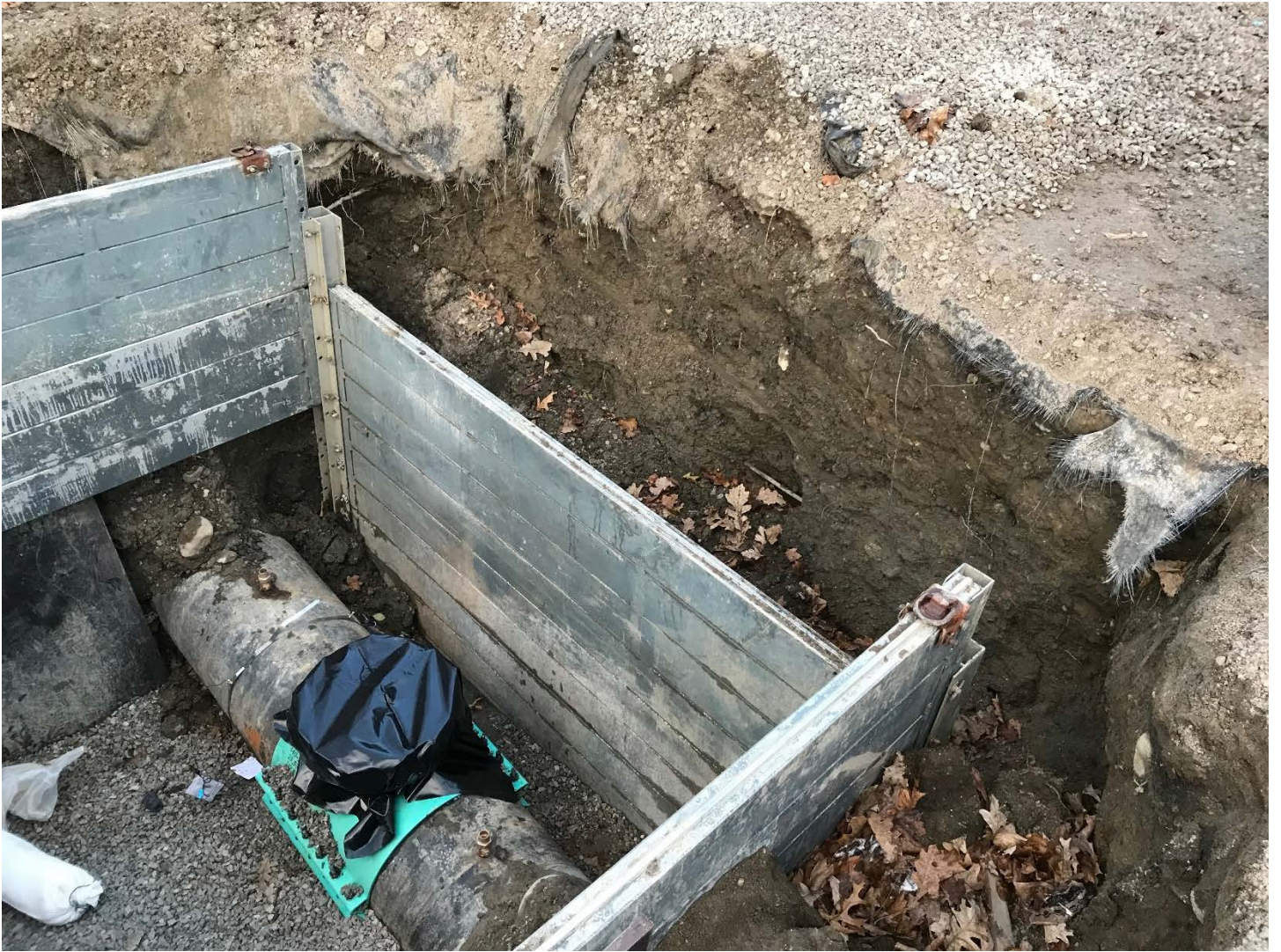
Figure 2 - 24" 1965 DI Main at Barton PS, Line Stop Fitting
