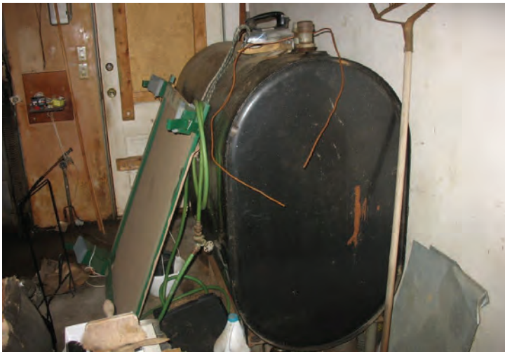
Viewing an approximate 275-gallon AST located in the garage of the house.
