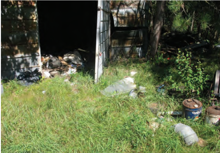
Facing east viewing the storage shed located south of the house.
