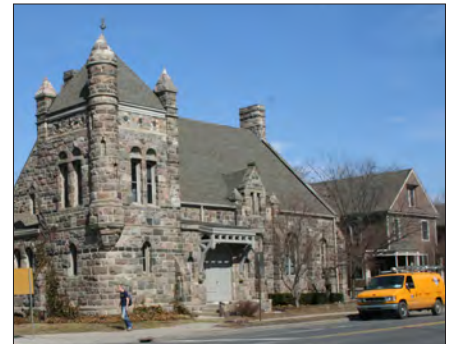
The Old Fourth Ward Historic District is primarily residential but does include a number of churches.
