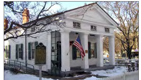
The Kempf House is a Greek Revival style structure in the Division Street Historic District.
