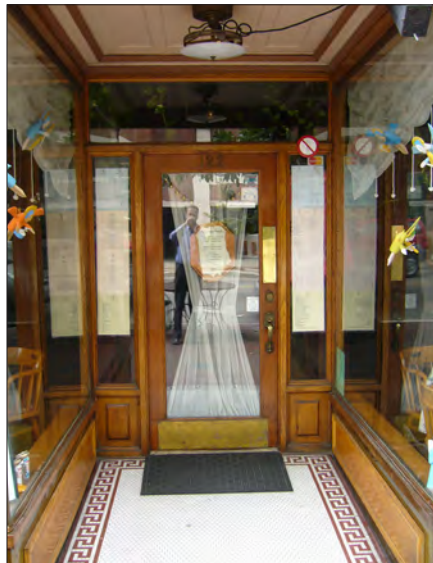
Many commercial storefronts in Ann Arbor feature recessed entries. In some cases, the entry floor and ceiling feature tile work or other decorative elements.
