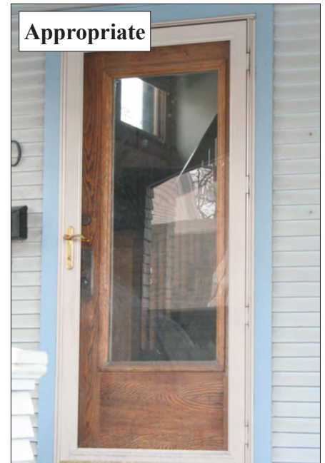
Retain, repair and maintain original doors.
