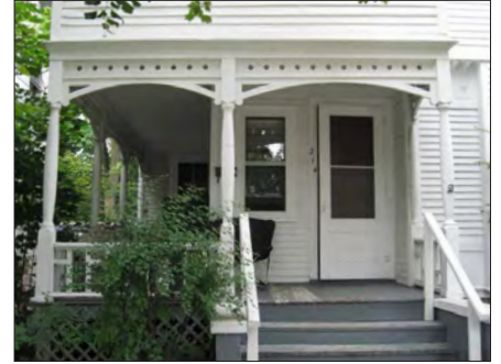
Porches contribute to the overall architectural style of a residential structure.
