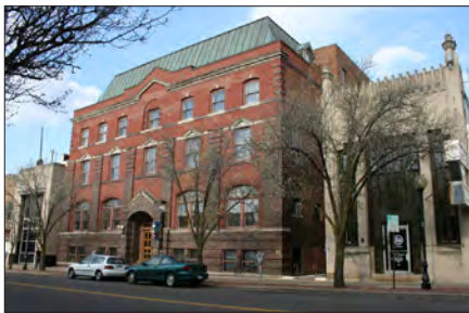
The 4th Avenue/Ann Street Historic District includes a variety of historic architectural styles.
