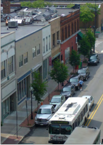
Historic commercial buildings such as those in the Main Street Historic District usually have flat roofs.
