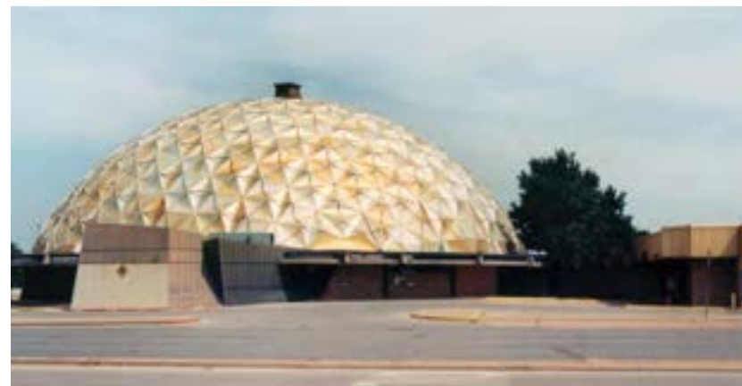
[13] The gold-colored, anodized aluminum geodesic dome of the former Citizen's State Bank in Oklahoma City, OK, built in 1958 and designed by Robert Roloff, makes this a distinctive mid-20th century building.
