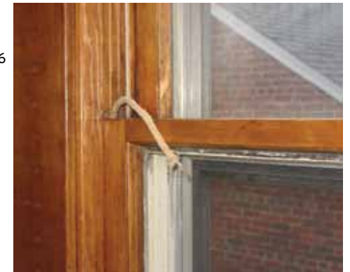
Not Recommended: [27] A broken sash cord can be repaired easily and does not justify replacement of the window.
