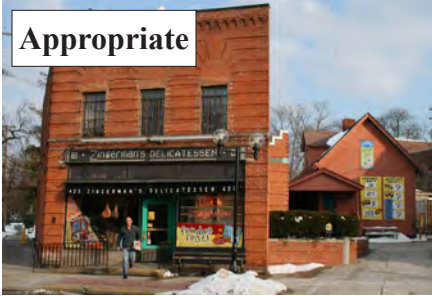
Design a new addition in a manner that makes clear what is historic and what is new.
