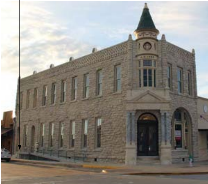
[53] This entrance ramp (right) is compatible with the historic character of this commercial building.
