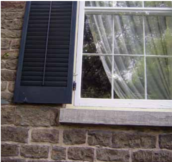
Recommended: [23-25] Historic exterior storm windows have been well maintained and continue to perform as intended.
