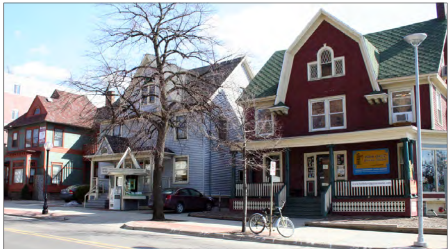
The roof shape and pitch is an important defining feature of a building's architecture.
