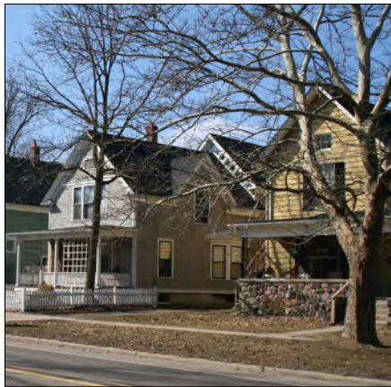
Many homes in the Old West Side Historic District have front facing gable roof forms.
