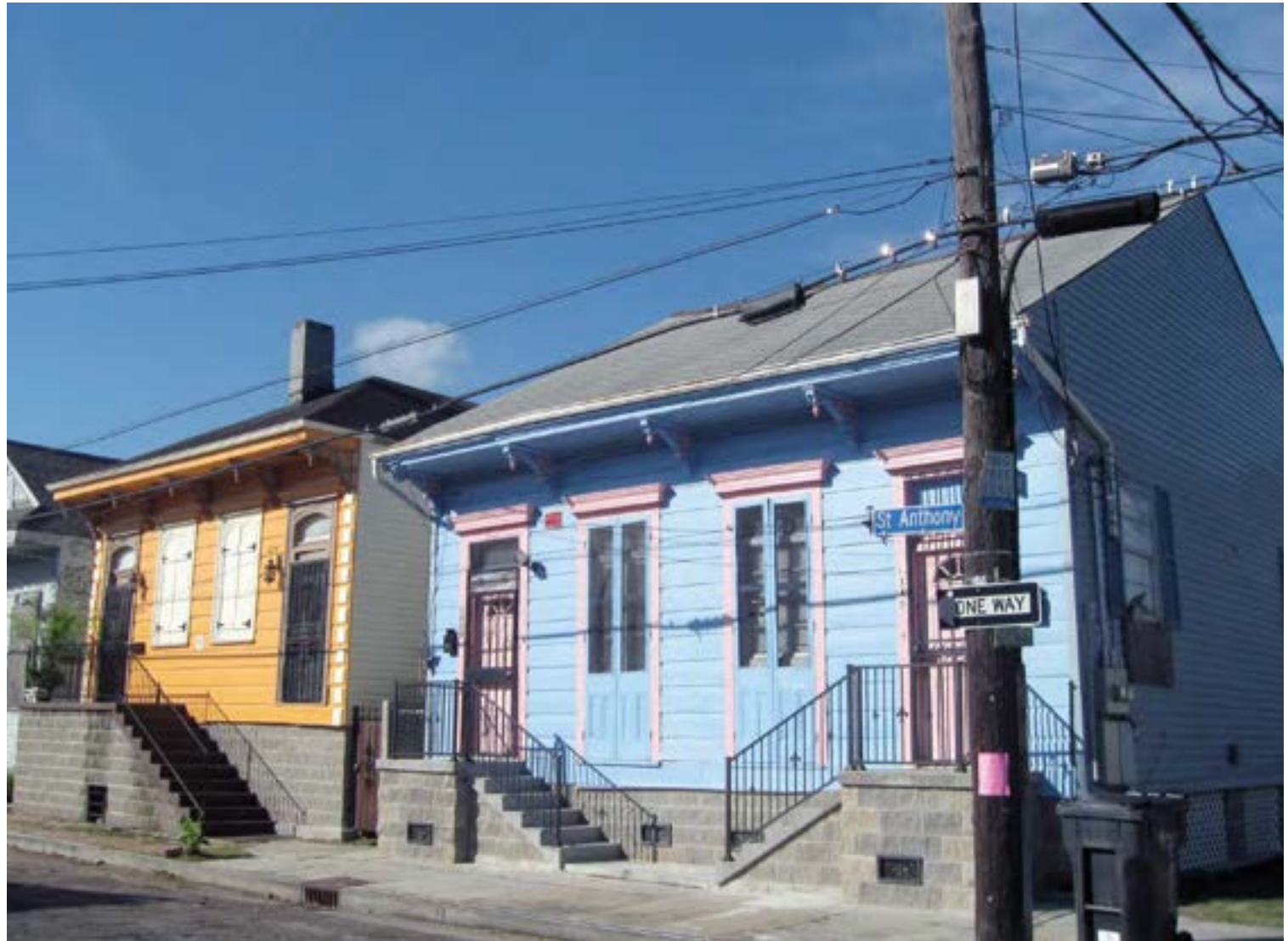
[60] In some instances, it may be necessary to elevate a historic building located in a floodplain to protect it. But this treatment is appropriate only if elevating the building will retain its historic character, including its relationship to the site, and its new height will be compatible with surrounding buildings if in a historic district. The house on the right, which has been raised only slightly, has retained its historic character. The house on the left has been raised several feet higher, resulting in a greater impact on the historic character of the house and the district.
