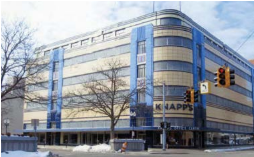
[7] (a) J.W. Knapp's Department Store, built 1937-38, in Lansing, MI, was constructed with a proprietary material named "Maul Macotta" made of enameled steel and cast-in-place concrete panels. Prior to its rehabilitation, a building inspection revealed that, due to a flaw in the original design and construction, the material was deteriorated beyond repair. The architects for the rehabilitation project devised a replacement system (b) consisting of enameled aluminum panels that matched the original colors (c). Photos and drawing (a-b): Quinn Evans Architects; Photo (c): James Haefner Photography.
