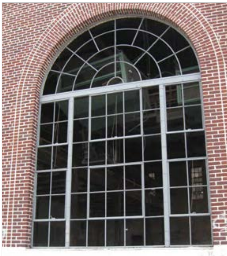
[12] This historic steel window has been cleaned, repaired, and primed in preparation for painting and reglazing.
