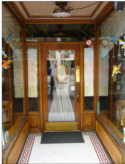
Many commercial storefronts in Ann Arbor feature recessed entries. In some cases, the entry floor and ceiling feature tile work or other decorative elements.
