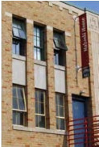
[21] The windows on the lower floor, which were too deteriorated to repair, were replaced with new steel windows matching the upper-floor historic windows that were retained.
