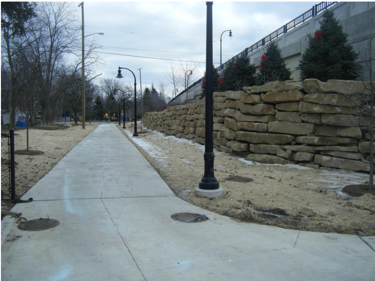
New walkway facing east at State Street
