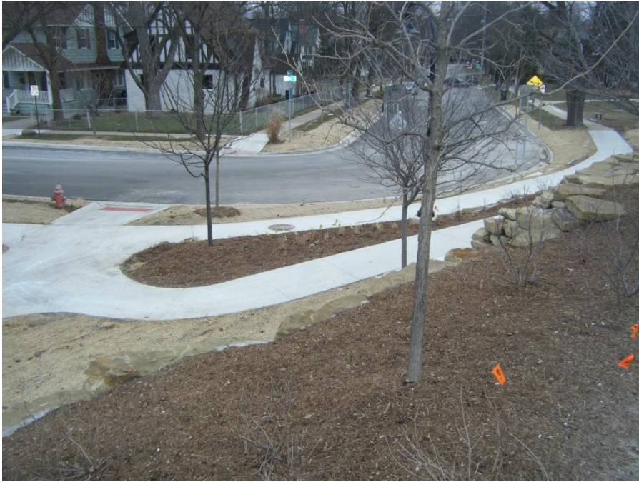
From Stadium Blvd. facing the White Street termination
