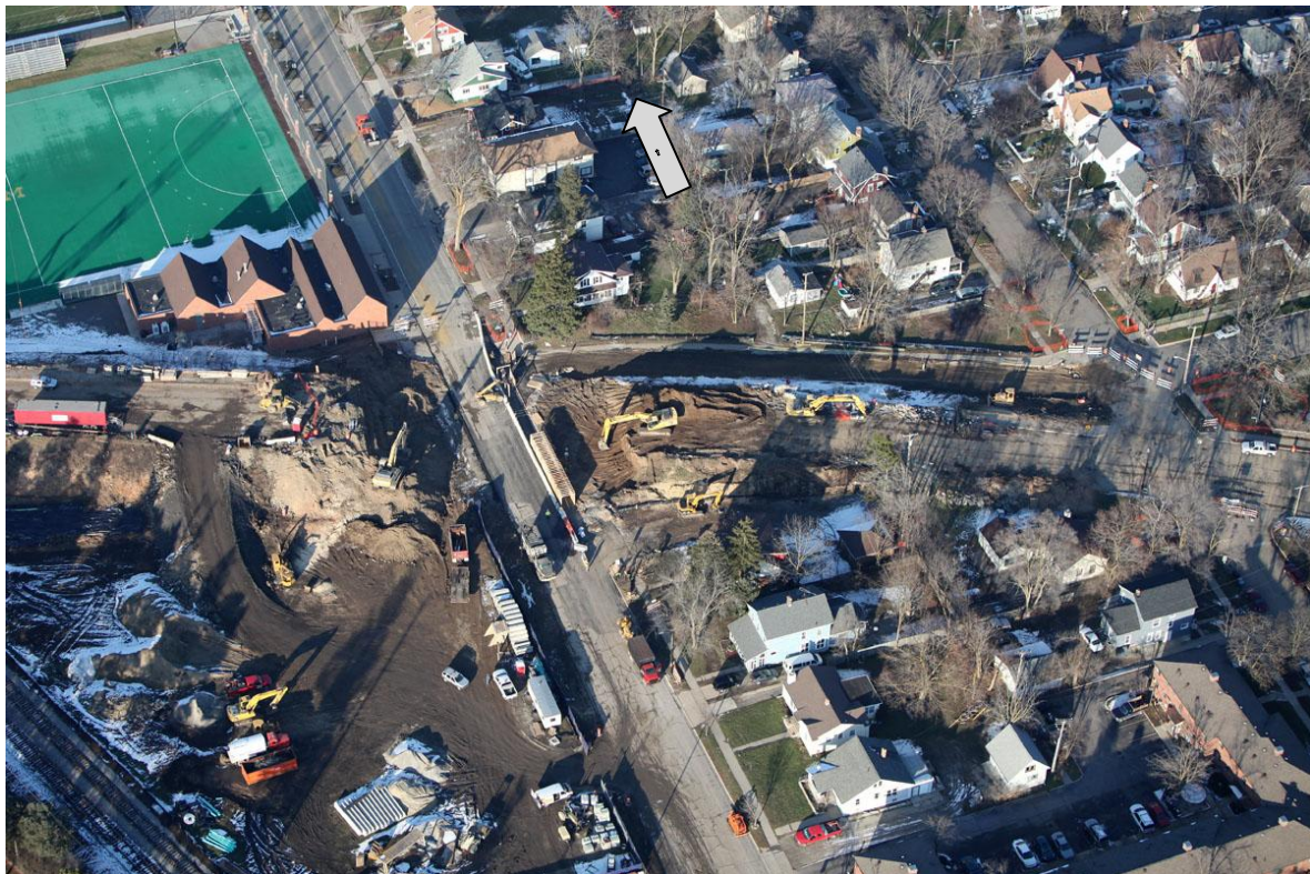
Photo of construction site December 2011
