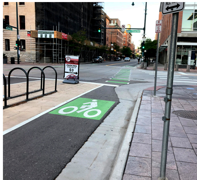
Raised Bike Lane in Denver, CO
