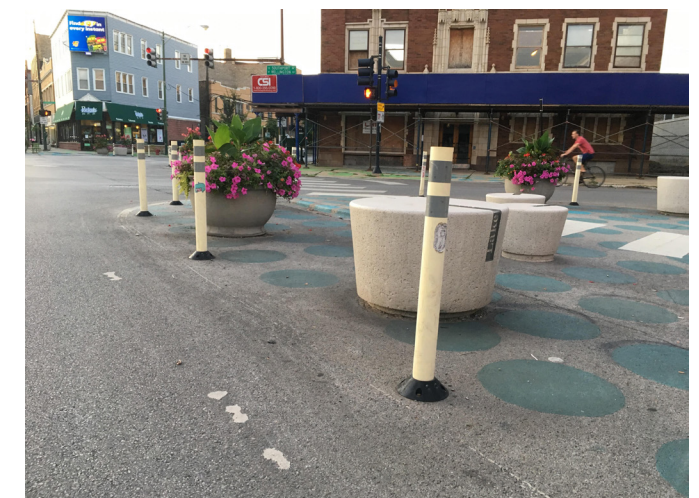
Flexible delineator posts
