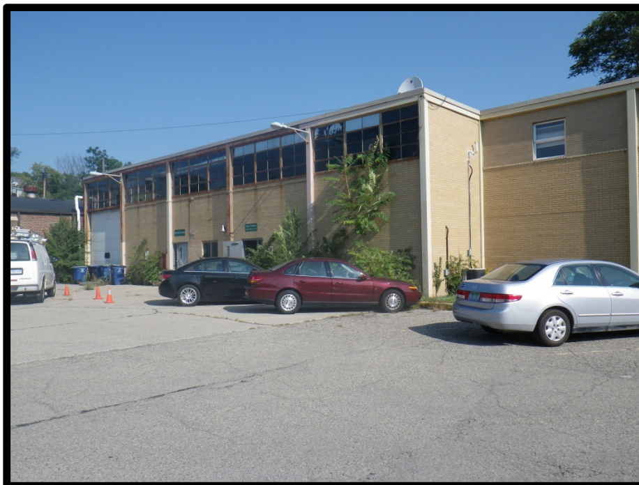
Looking northwest at the northern section of the maintenance building
