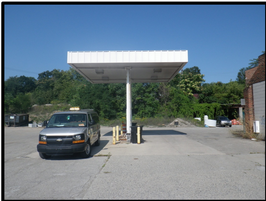
Looking west at the former fuel dispenser island
