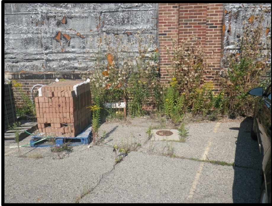
A monitoring well located east of the maintenance building
