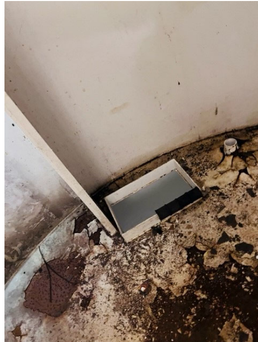
Openings Field verify dimensions – picture 2
