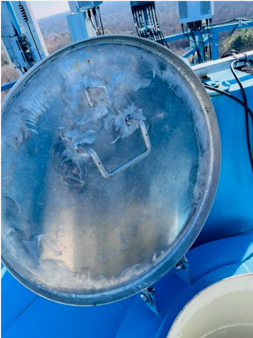
North Campus hatch to be replace with an aluminum hatch to match Manchester tank's hatch – picture 3
