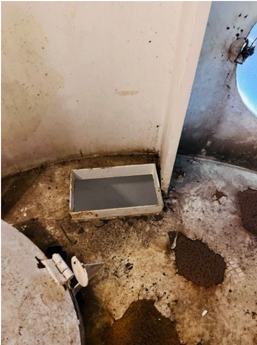
Openings Field verify dimensions – picture 1
