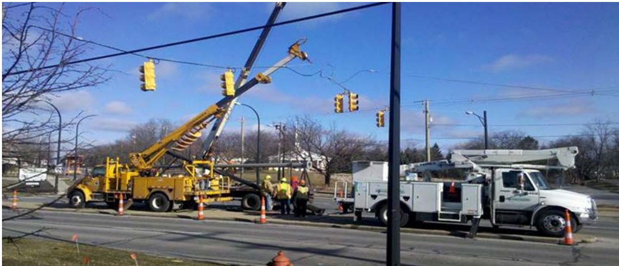
Washtenaw Ave & Stadium Blvd Utility Work
