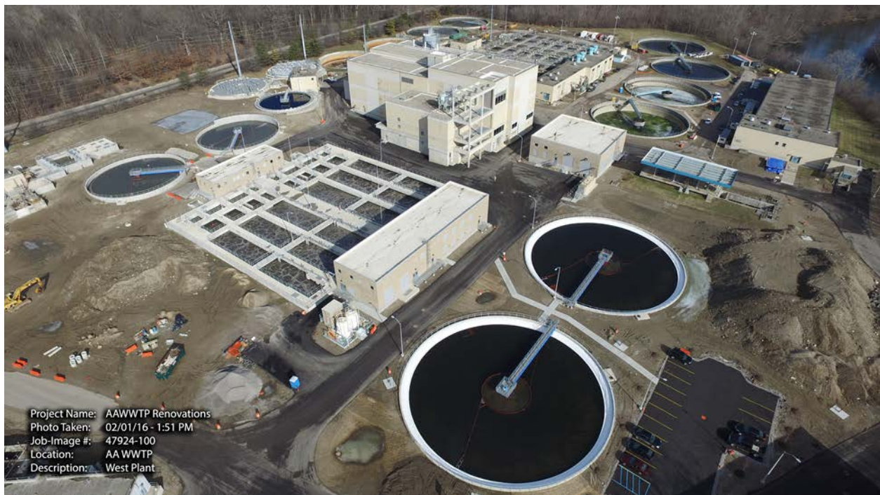
Wastewater Treatment Plant Facilities Renovations Project
