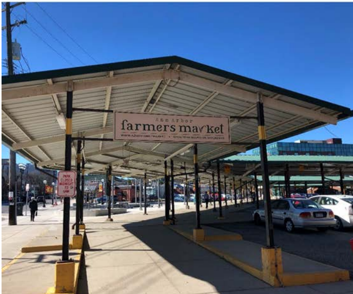
Existing Metal Building Canopy – north end along Detroit Street
