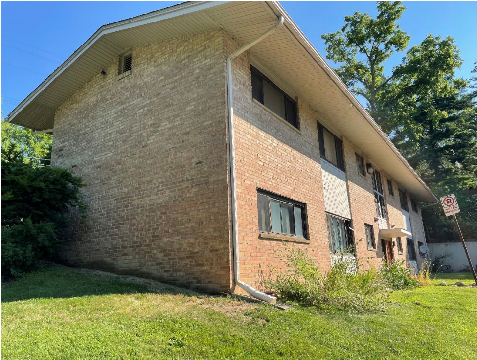
Photograph 5: View of the west/south 1504 building elevation.
