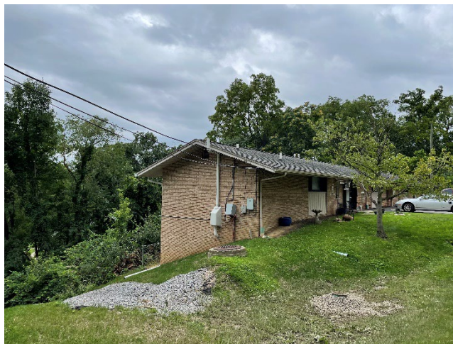
Photograph 11: View of building 1508 (note radon system venting).
