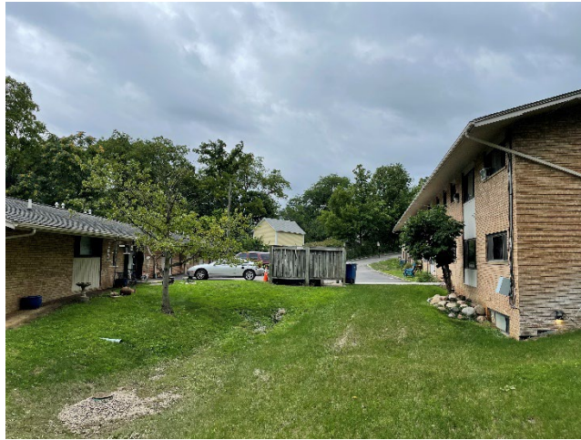
Photograph 10: View of building 1508 (left) and 1506 (right).
