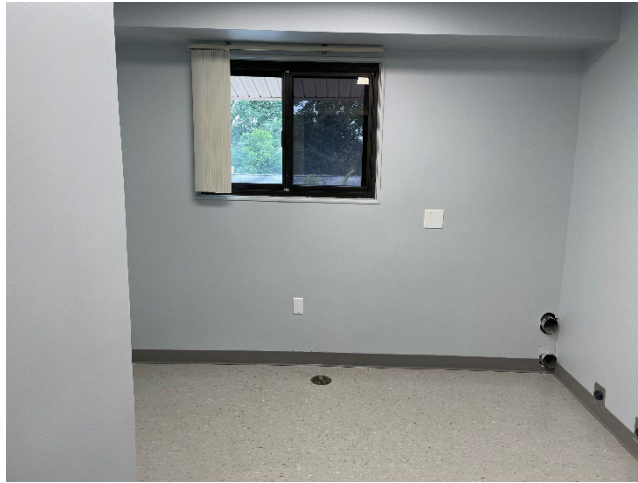
Photograph 19: Interior view, future community laundry room.
