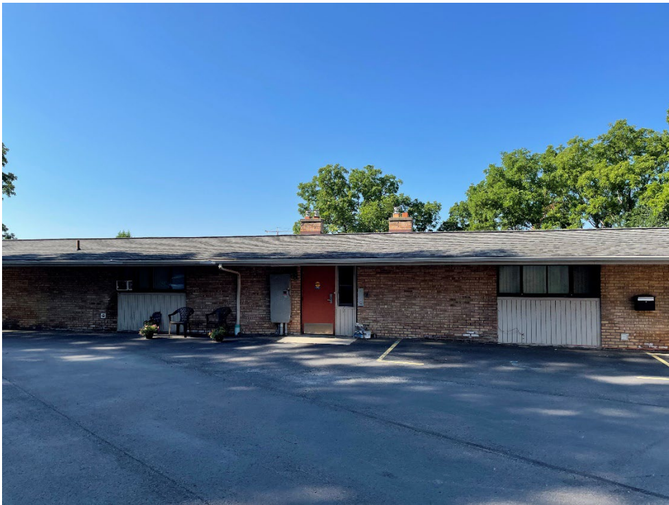
Photograph 6: View of the central apartment building 1506 and adjoining parking.
