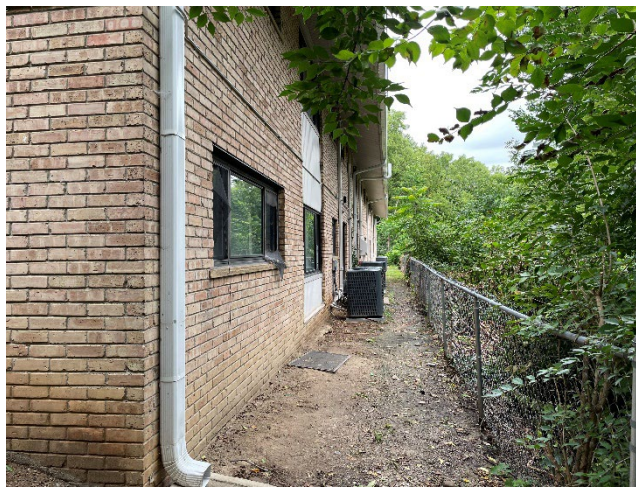
Photograph 14: Rear of building 1508 (southern building elevation).
