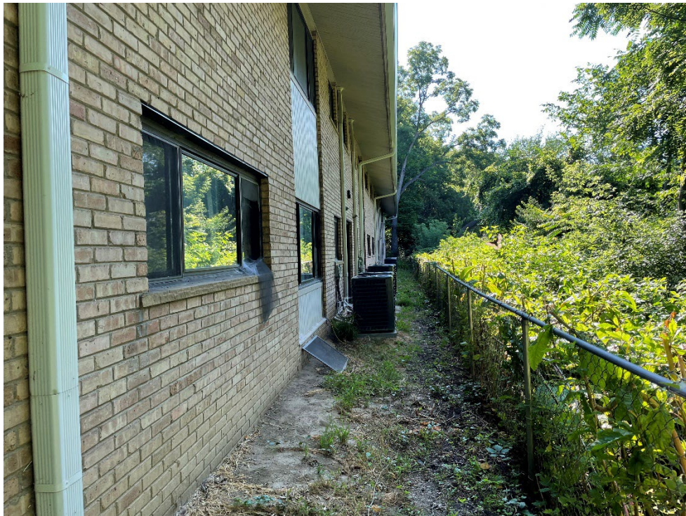
Photograph 14: Rear of building 1508 (southern building elevation).
