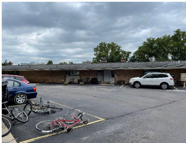
Photograph 5: View of the central apartment building 1506 and adjoining parking.
