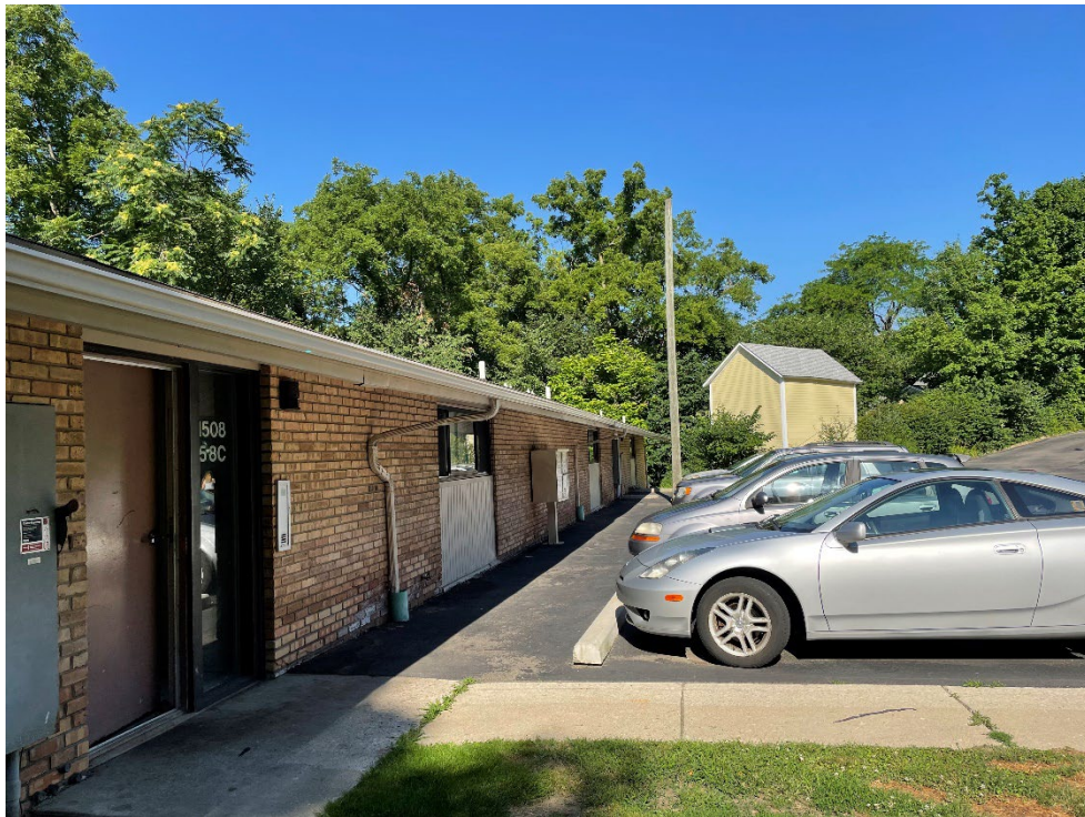
Photograph 12: View of the north building elevation of 1508.
