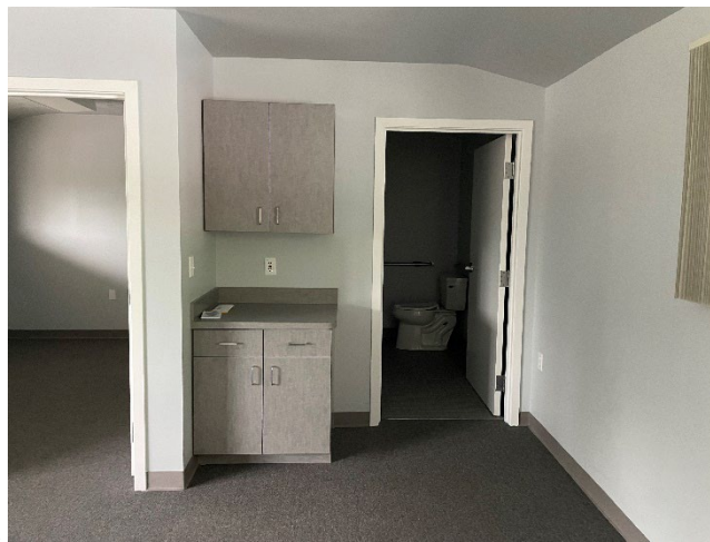
Photograph 20: Interior view, future community room.
