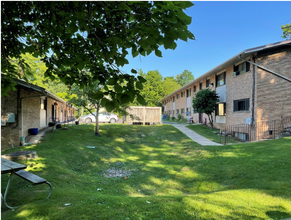
Photograph 10: Near the east corner of the property looking west across the site.
