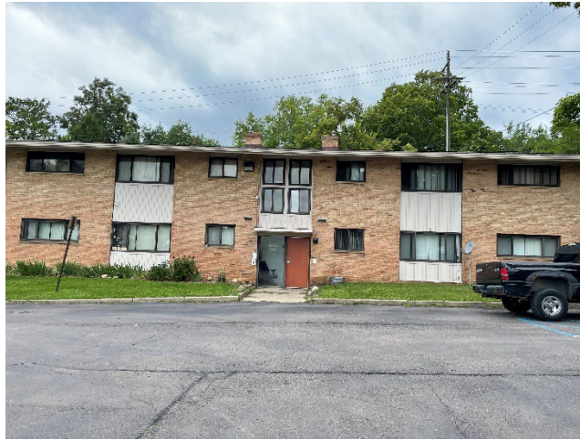
Photograph 4: View of the west/south 1504 building elevation and adjoining parking area.
