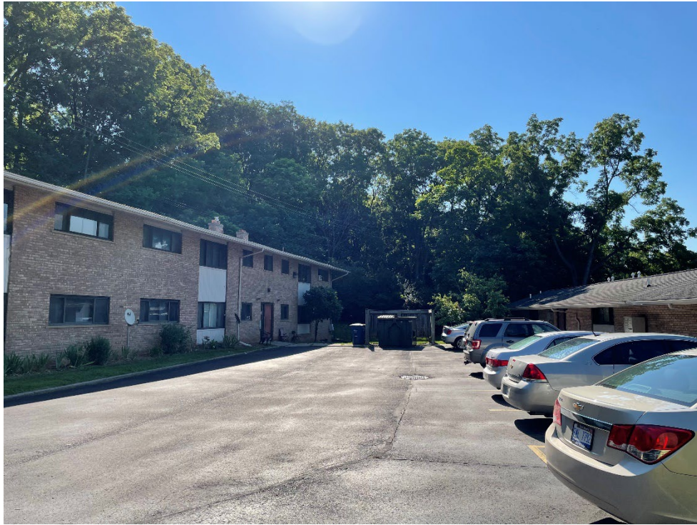
Photograph 13: Looking east across the parking area between 1506 (left) and 1508 (right).
