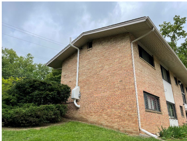
Photograph 3: Side elevation (south) of building 1504 (note radon system venting).
