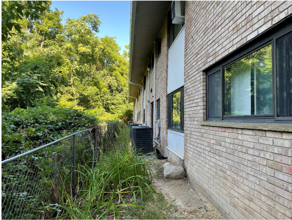
Photograph 11: Looking west across the rear of building 1508 (south building elevation).
