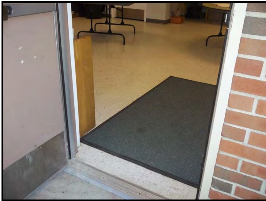
PHOTOGRAPH NO. 19: VIEW OF TYPICAL EXISTING FLOORING
