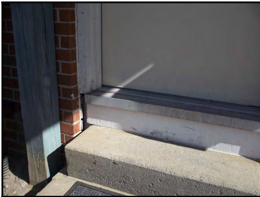
PHOTOGRAPH NO. 20: TYPICAL VIEW OF CONCRETE STEP TO UNIT ENTRANCE
