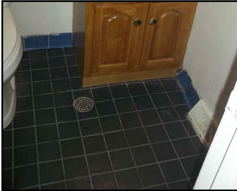
PHOTOGRAPH NO. 15: TYPICAL VIEW OF FLOORING IN TENANT UNIT BATHROOMS
