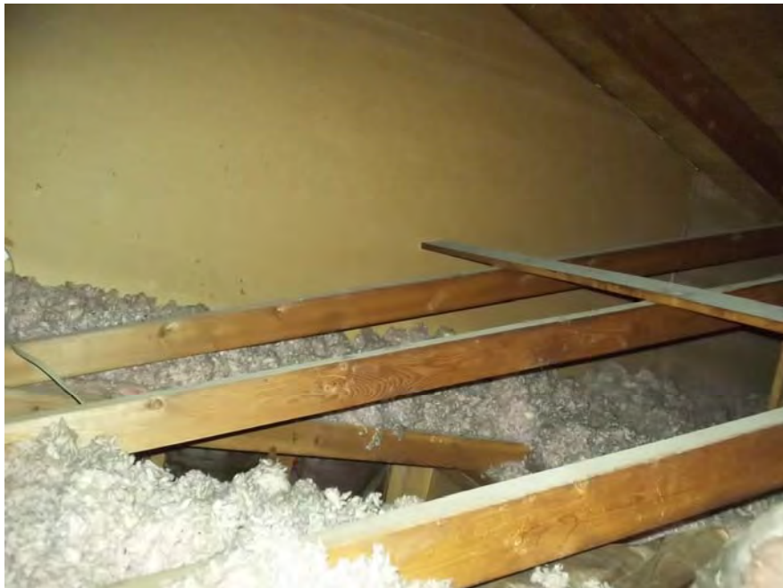
PHOTOGRAPH NO. 8: TYPICAL VIEW OF ATTIC INSULATION IN SUBJECT BUILDINGS
