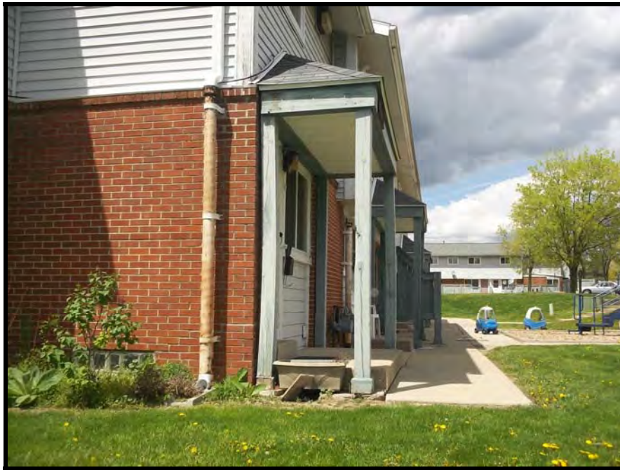
PHOTOGRAPH NO. 7: TYPICAL VIEW OF PORCHES ASSOCIATED WITH TENANT UNITS
