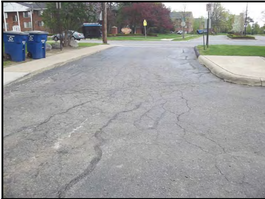
PHOTOGRAPH NO. 22: VIEW OF ASPHALT PAVEMENT IN PARKING LOT
