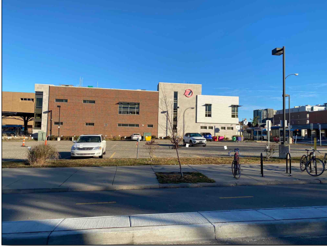
Looking North Across Central Region of the Site from E. William Street
