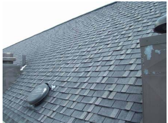
Photo #6: Pitched roof detail
