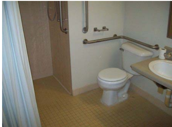
Photo #28: Accessible unit bathroom
