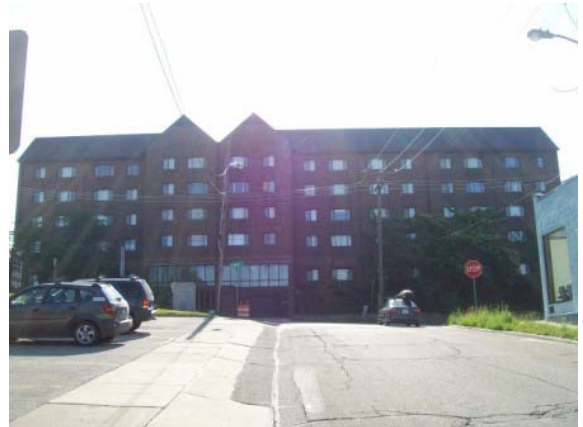
Photo #4: Rear elevation of building
