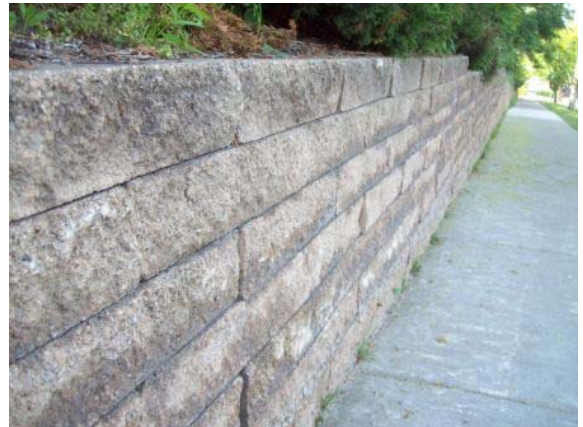
Photo #76: Retaining wall at west property line
