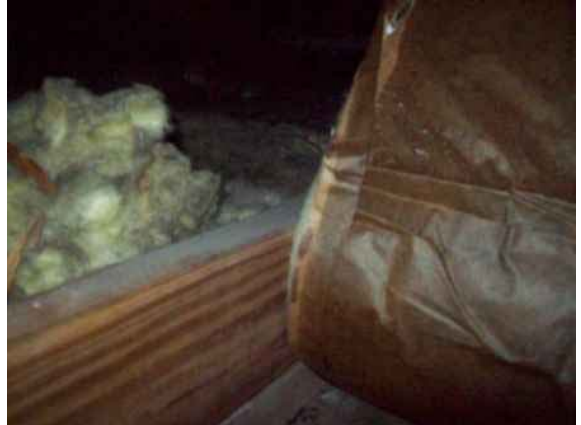
Photo #8: Batt insulation in attic
