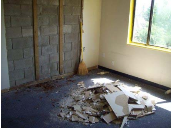
Photo #31: Down unit undergoing repairs
