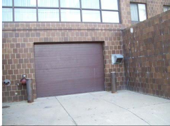
Photo #14: Overhead service door
