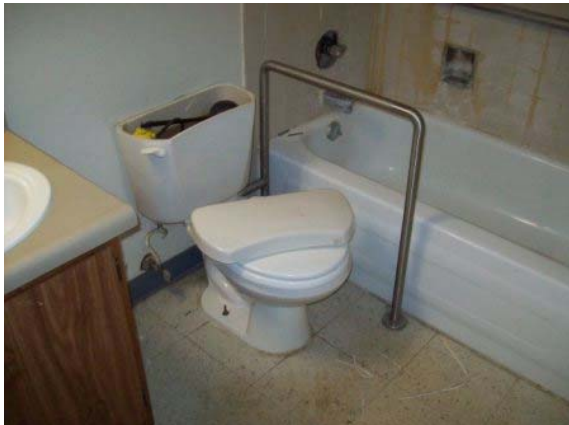
Photo #27: Apartment unit bathroom
