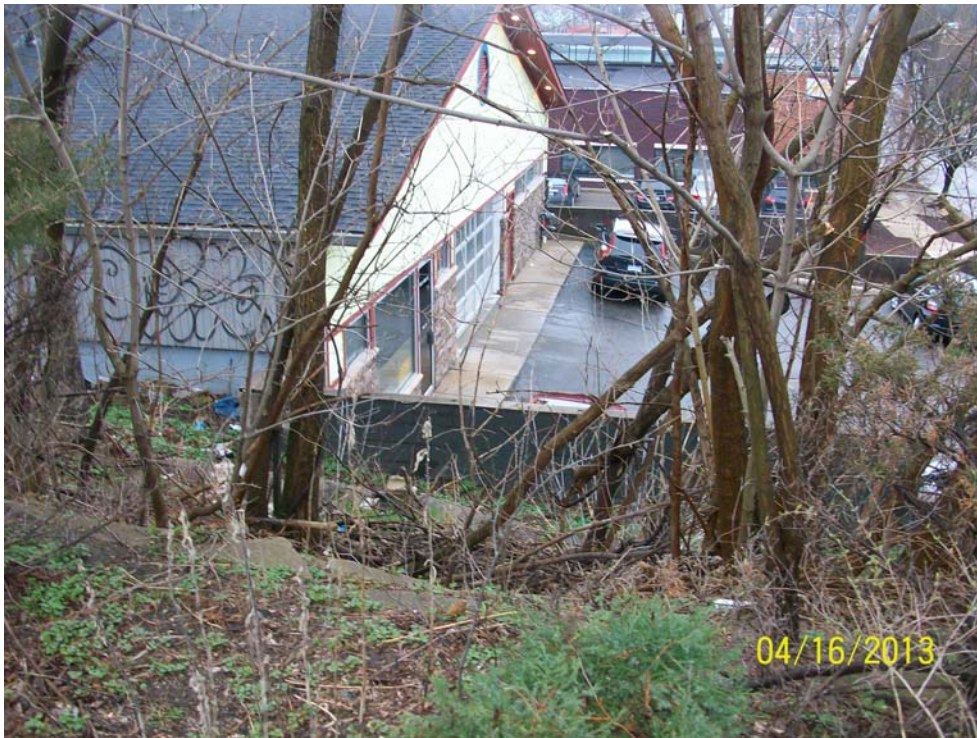
Photograph 26: South adjoining auto repair, view facing south.
