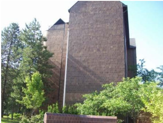
Photo #3: Side elevation of building
