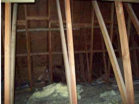
Photo #7: Roof structure in attic
