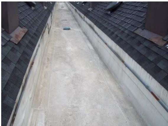
Photo #9: Flat roof finish
