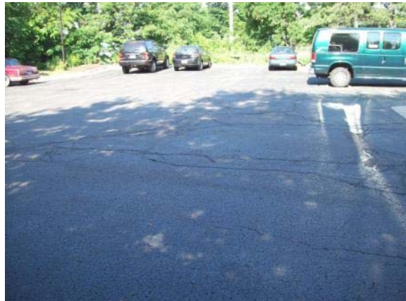
Photo #16: Back parking area
