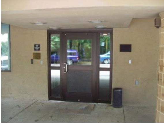
Photo #13: Main entrance doors
