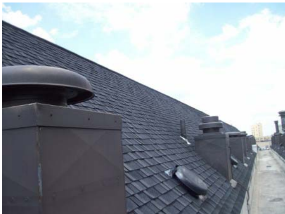
Photo #5: Roof overview
