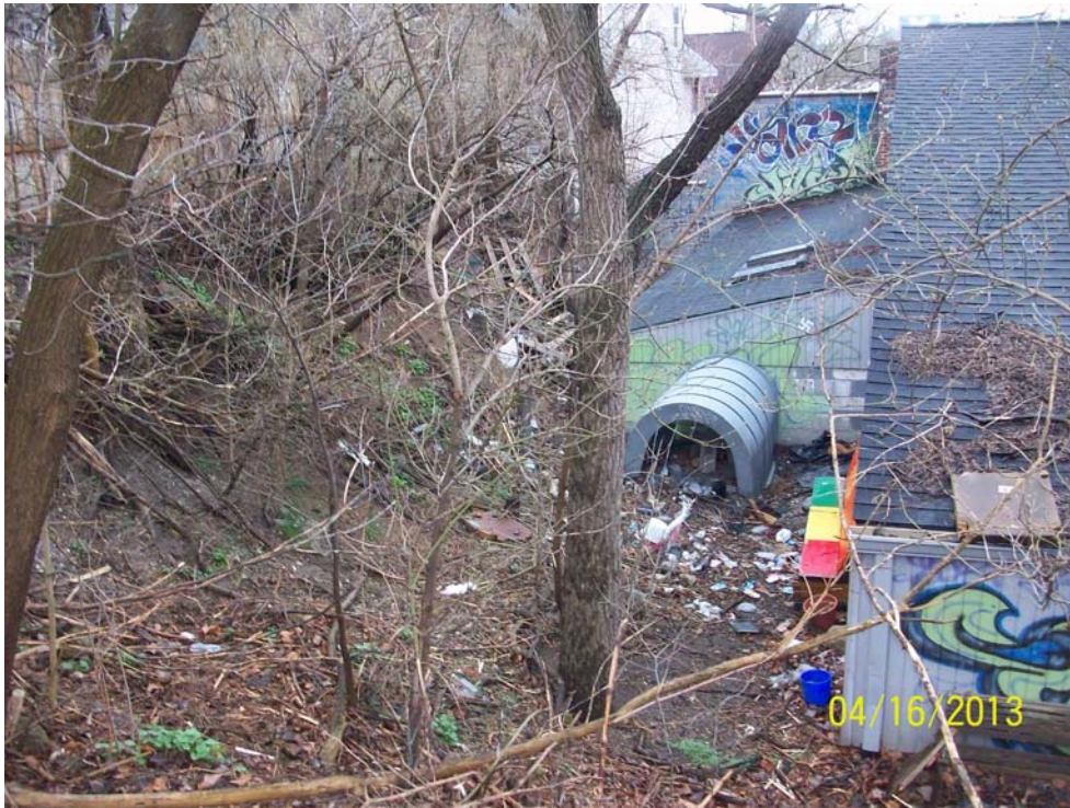
Photograph 27: South adjoining auto repair, view facing south.
