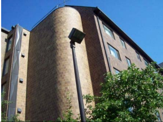
Photo #73: Exterior pole-mounted lighting
