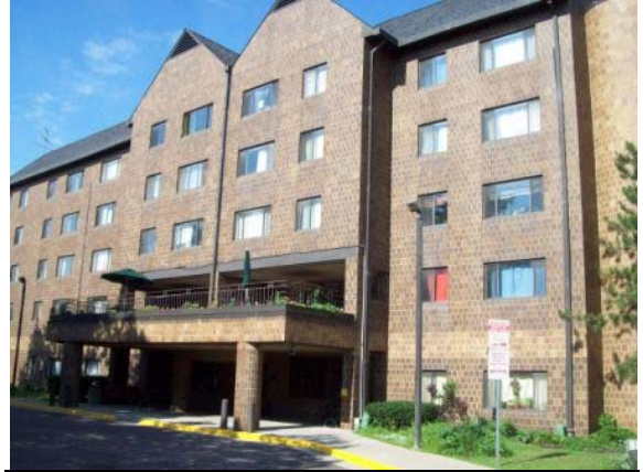
Photo #2: Front elevation of building
