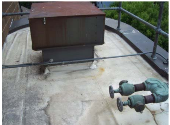
Photo #10: Flat roof membrane detail
