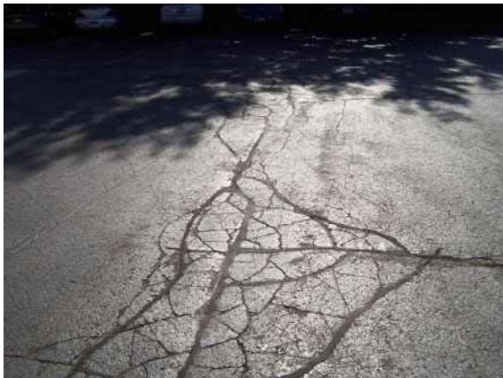
Photo #17: Pavement detail
