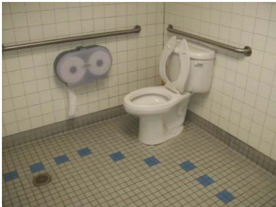
Photo #23: Common area restroom
