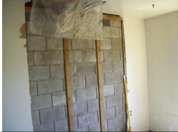
Photo #32: Wall repair at down unit
