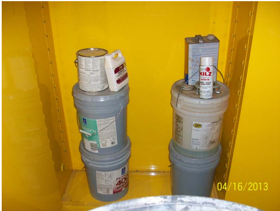
Photograph 20: Paint storage observed in the basement of the building.
