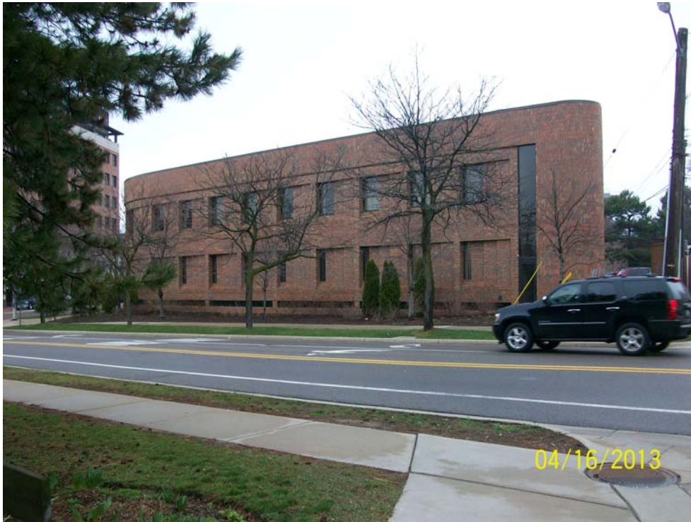
Photograph 25: North adjoining commercial building, view facing north across Packard Street.
