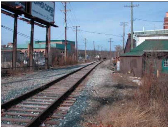
AARR tracks looking North to the embankment
