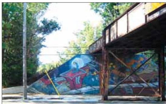
AARR tressle bridge
