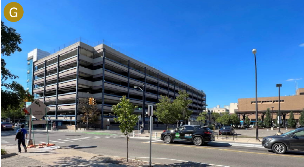
Fourth & William Parking Garage
