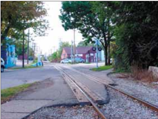
The mixing of track, street and sidewalk
