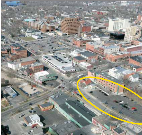
Parking lot at First and William Streets
