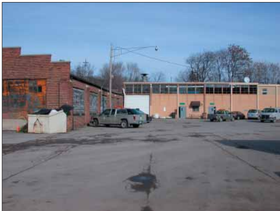
Existing buildings in the flood fringe
