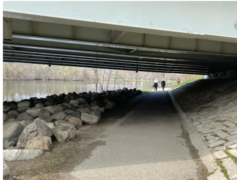
BRIDGE UNDERPASS - EXISTING 8' WIDE ASPHALT PATH. NEW 10' WIDE PATH WILL EXTEND TO THE SOUTH (LEFT).
