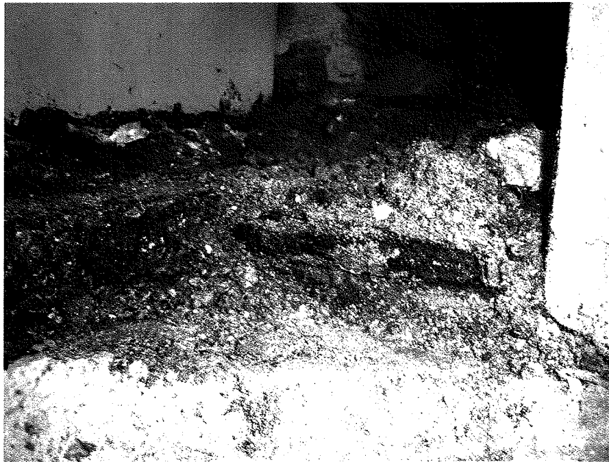
Debris, Surface Rusting, Minor Deterioration at East Abutment, South Beam Bearing
