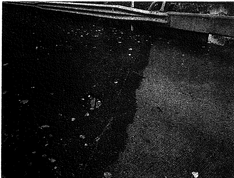
Cracking and Pothole near East Reference Line
