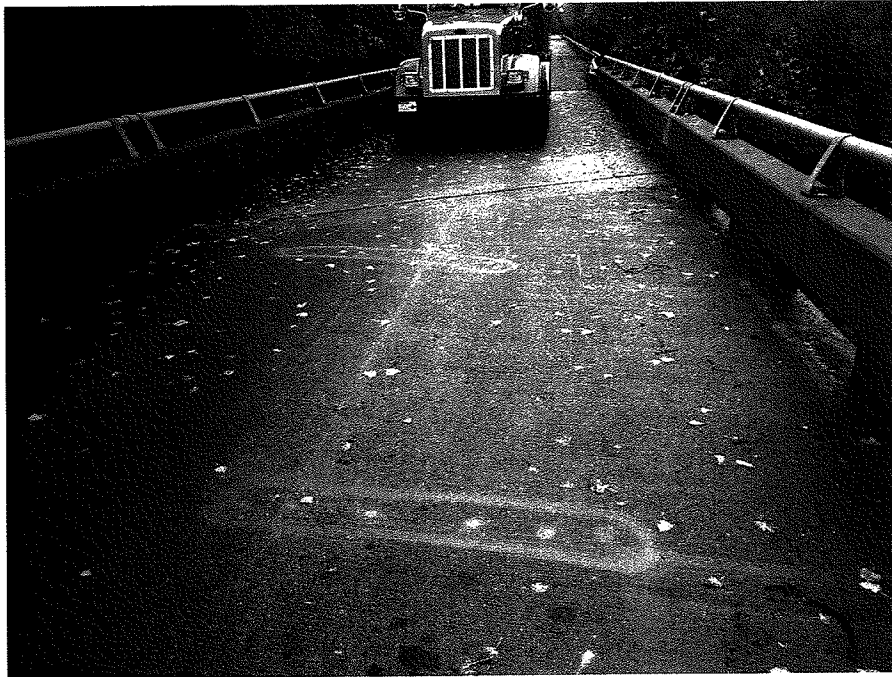
Photograph No. 11 West Half of East Span Looking West
