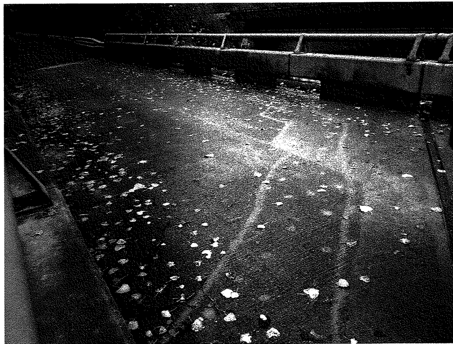
Photograph No. 14 Bridge Railing in Good Condition (North Shown)
