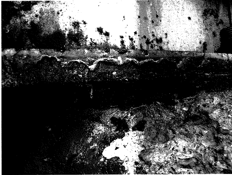
Photograph No. 39 Spalling at South Fascia Bearing at West Side of Pier
