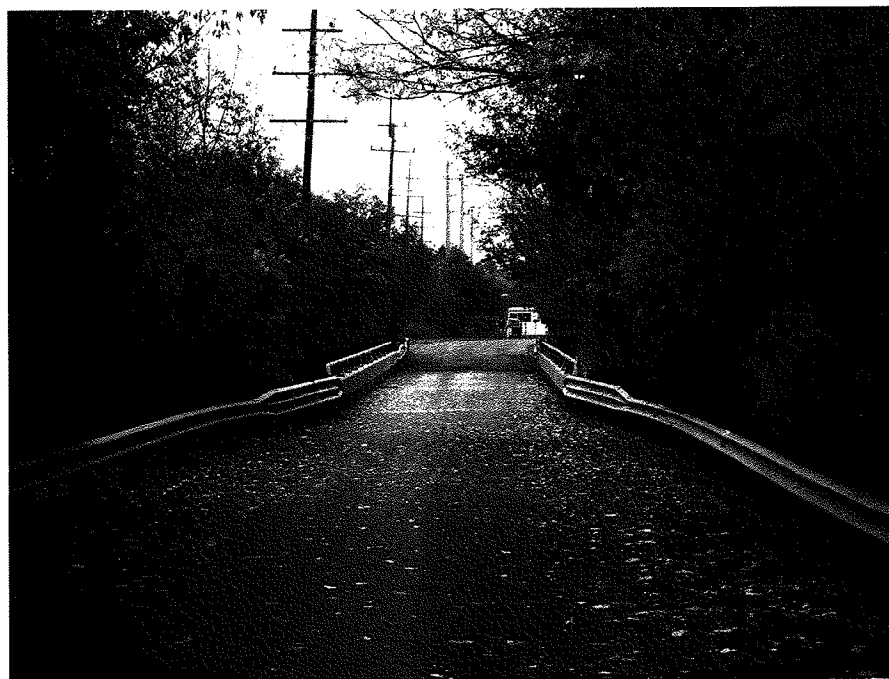
Photograph No. 6 West Approach Looking East
