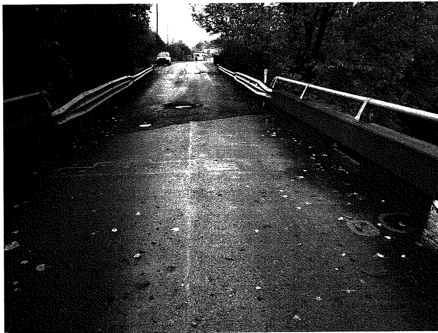
Photograph No. 12 East Half of East Span Looking East
