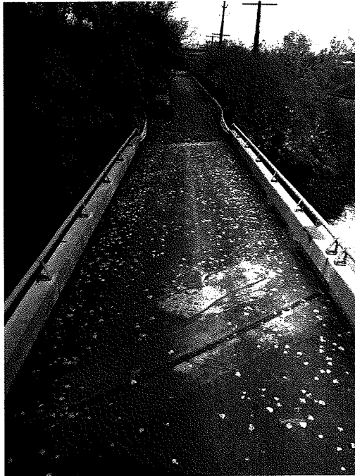
Photograph No. 7 West End of the Deck Looking West
