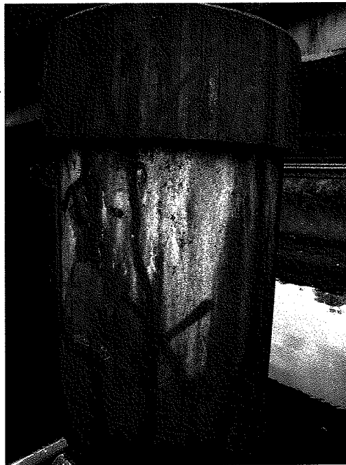
Photograph No. 40 Delaminations and Cracking on North End of Pier
