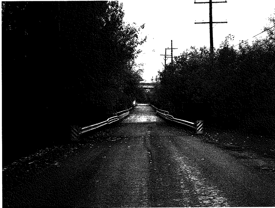
Photograph No. 3 East Approach Looking West
