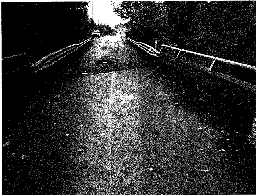
Photograph No. 4 East Approach Looking East
