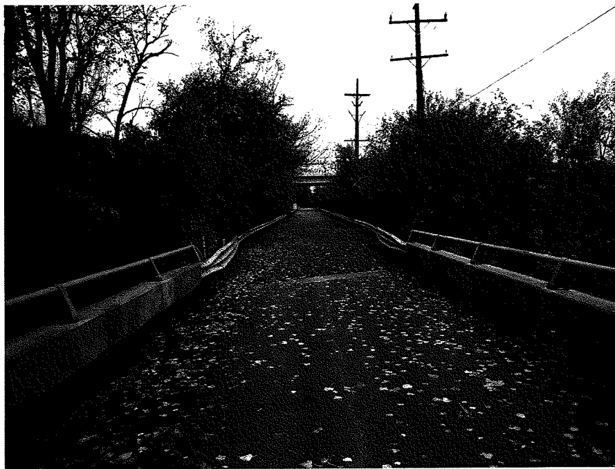
Photograph No. 5 West Approach Looking West
