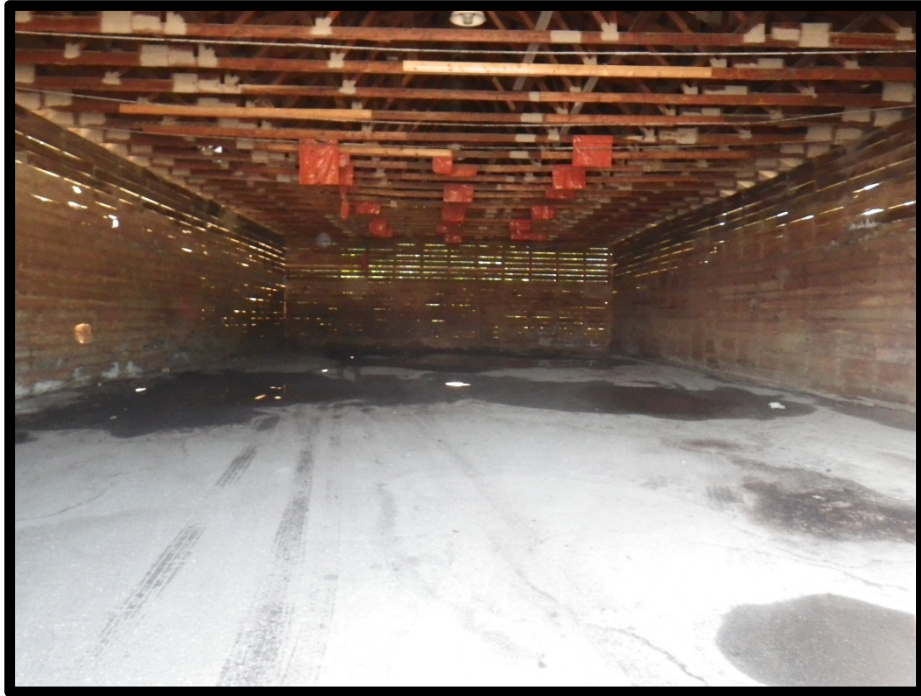
Looking south inside the wooden salt storage barn
