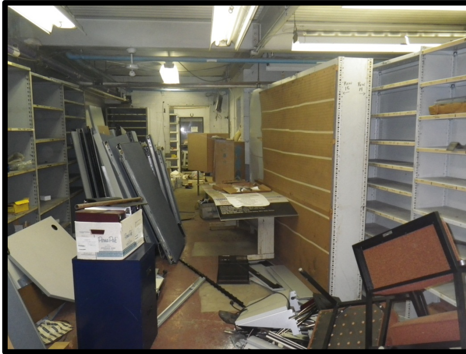
Inside the offices of the maintenance building
