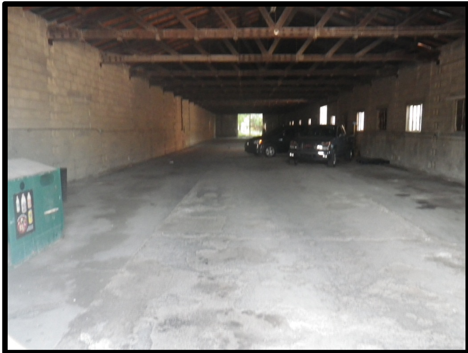
Looking south inside the garbage barn
