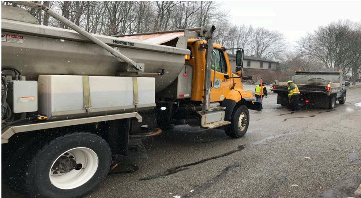
Bluett Road Pothole Patching
