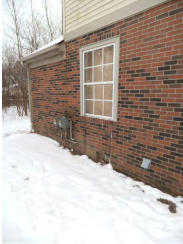
Photo 11: Exterior view of typical window
