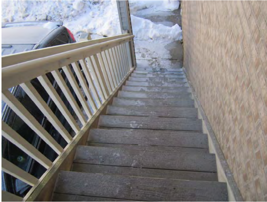
PHOTOGRAPH NO. 7: TYPICAL VIEW OF DECK COMPONENTS
