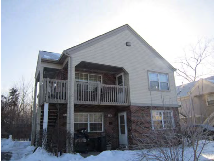
PHOTOGRAPH NO. 1: TYPICAL VIEW OF TENANT UNIT BUILDING
