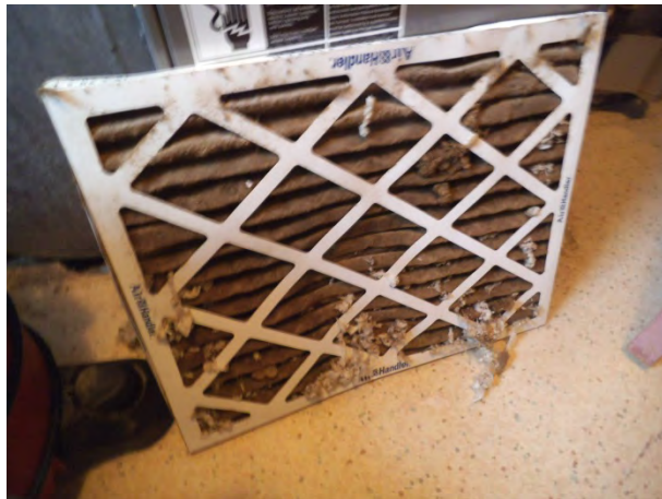
Photo 13: Filter from furnace in need of replacement
