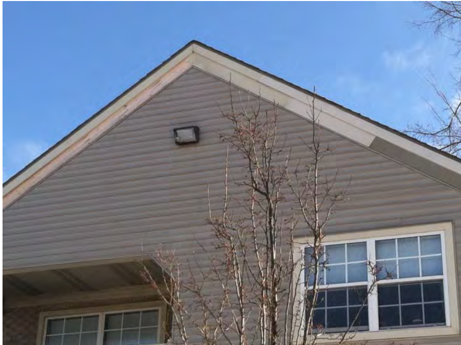
PHOTOGRAPH NO. 6: TYPICAL VIEW OF ROOFS (SOUTH FACING)
