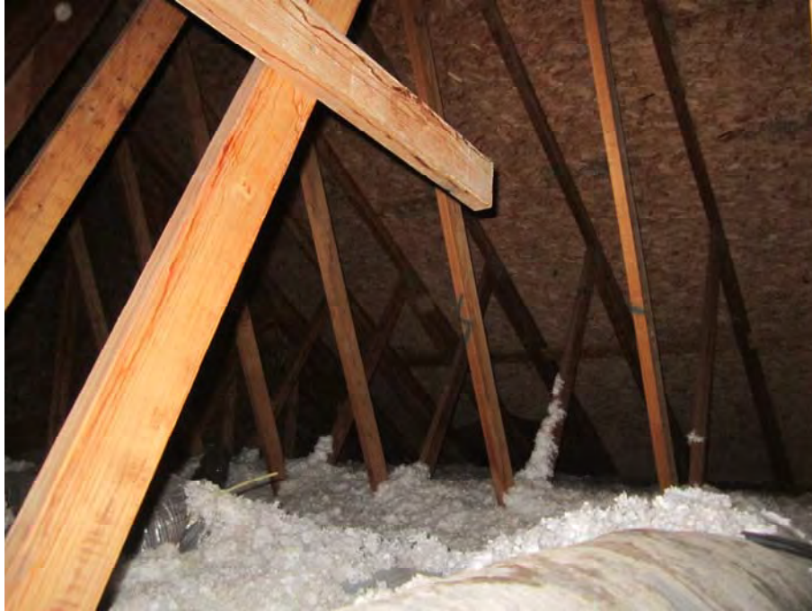
PHOTOGRAPH NO. 13: TYPICAL VIEW OF ATTIC SPACE
