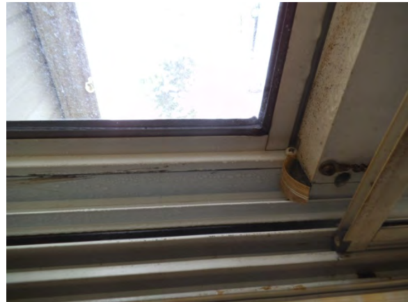
Photo 10: Condensation on the interior of windows
