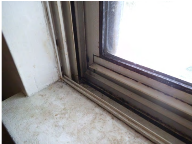
Photo 4: Typical Window Frame
