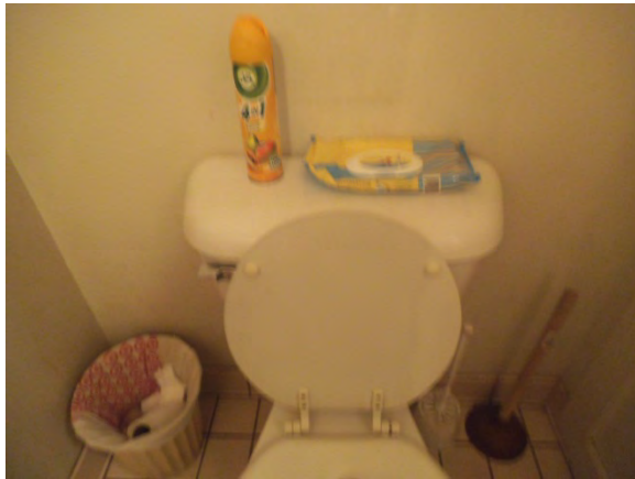
Photo 9: Typical bathroom toilet
