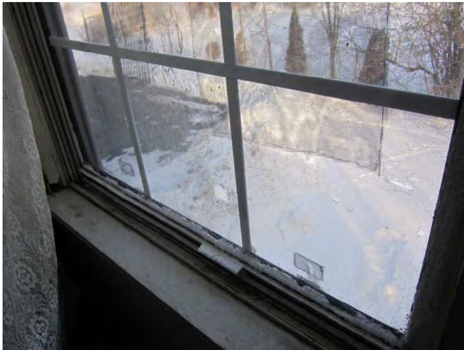
PHOTOGRAPH NO. 16: TYPICAL INTERIOR VIEW OF TENANT UNIT WINDOWS
