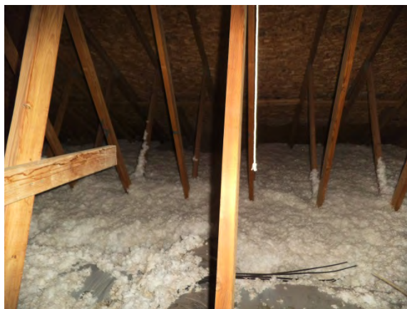
Photo 11: Attic framing and insulation
