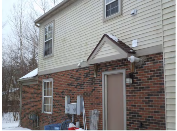
Photo 2: Side Entrance to Complex
