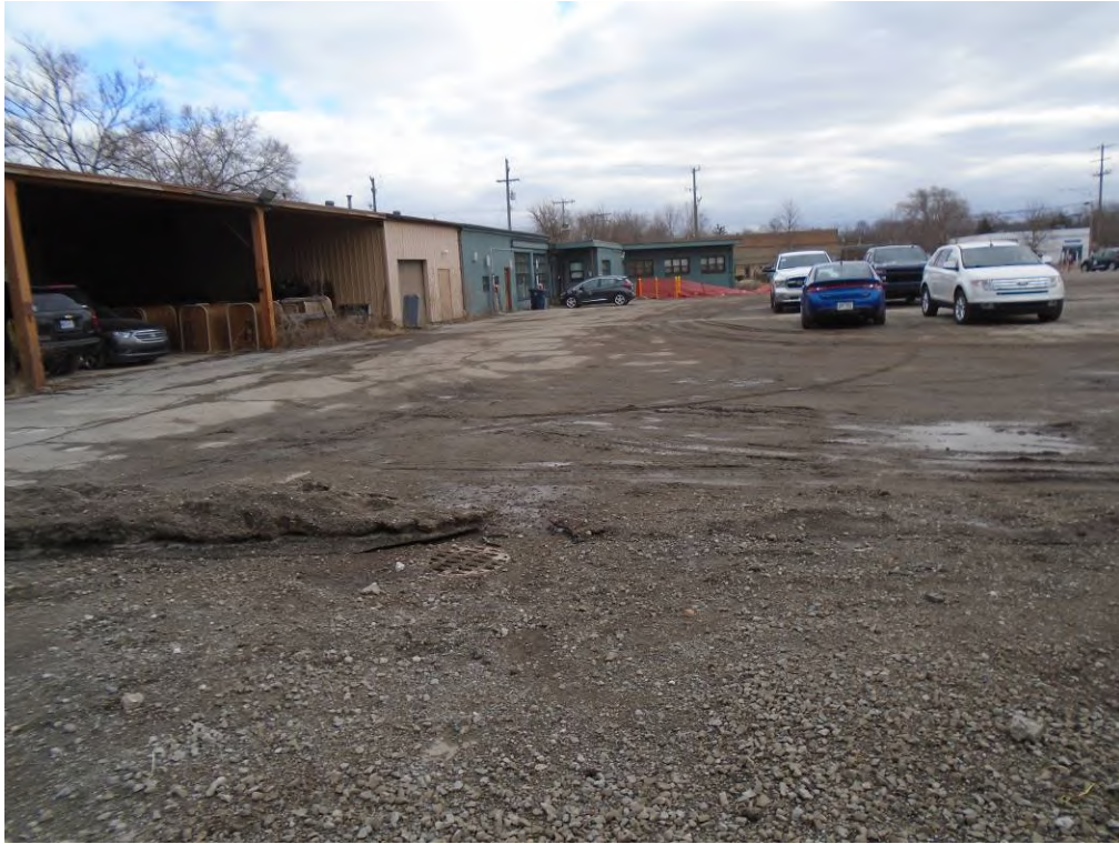
Photo 5: View of the southern portion of the 2000 South Industrial Highway subject property building, facing east. Note the secure unassessed furniture warehouse space east of the open storage area.
