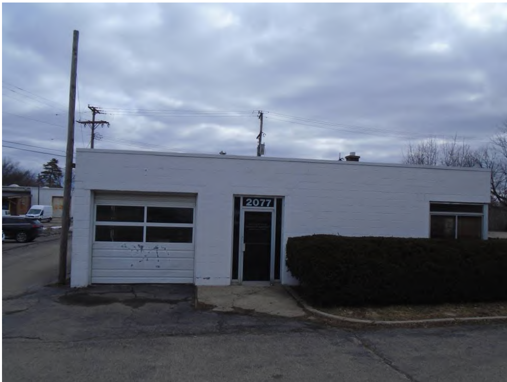
Photo 48: View of western adjoining property across railroad tracks Sure-Flo Fittings/Perfection Sprinklers (2077 S. State).
