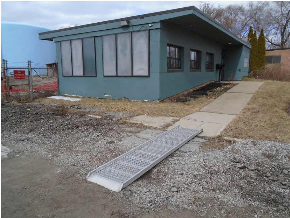
Photo 2: View of the eastern portion of the 2000 South Industrial Highway subject property building, facing north. Note the disturbed soil/asphalt parking lot for drainage.
