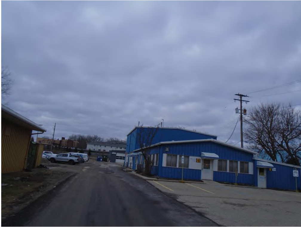
Photo 45: View of southern adjacent property Multi-Tenant Commercial (2200 S. Industrial).
