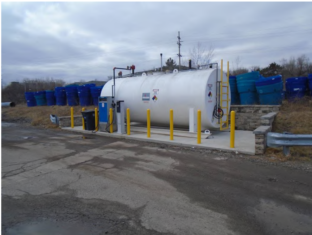
Photo 18: View of 15,000-gallon gasoline AST, facing southwest.
