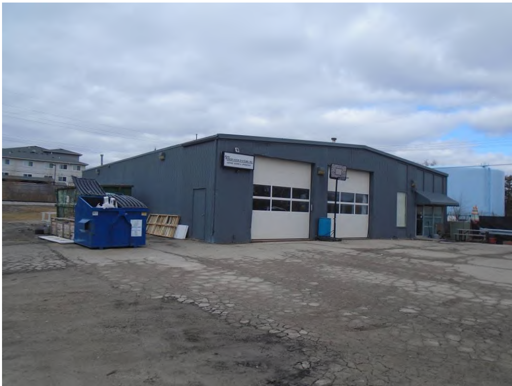
Photo 46: View of southern adjacent property Multi-Tenant Commercial – Ann Arbor Door Systems (2200 S. Industrial).
