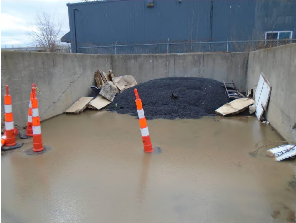
Photo 35: View of the southern portion of the subject property, flooded drain commission storage, facing south.
