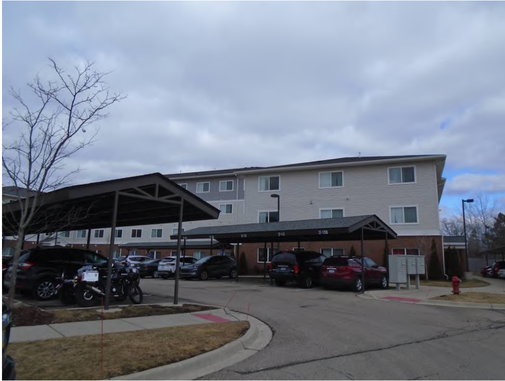
Photo 51: View of western adjoining property across railroad tracks State Street Village Apartments – Bldg #2227 (2221 S. State).
