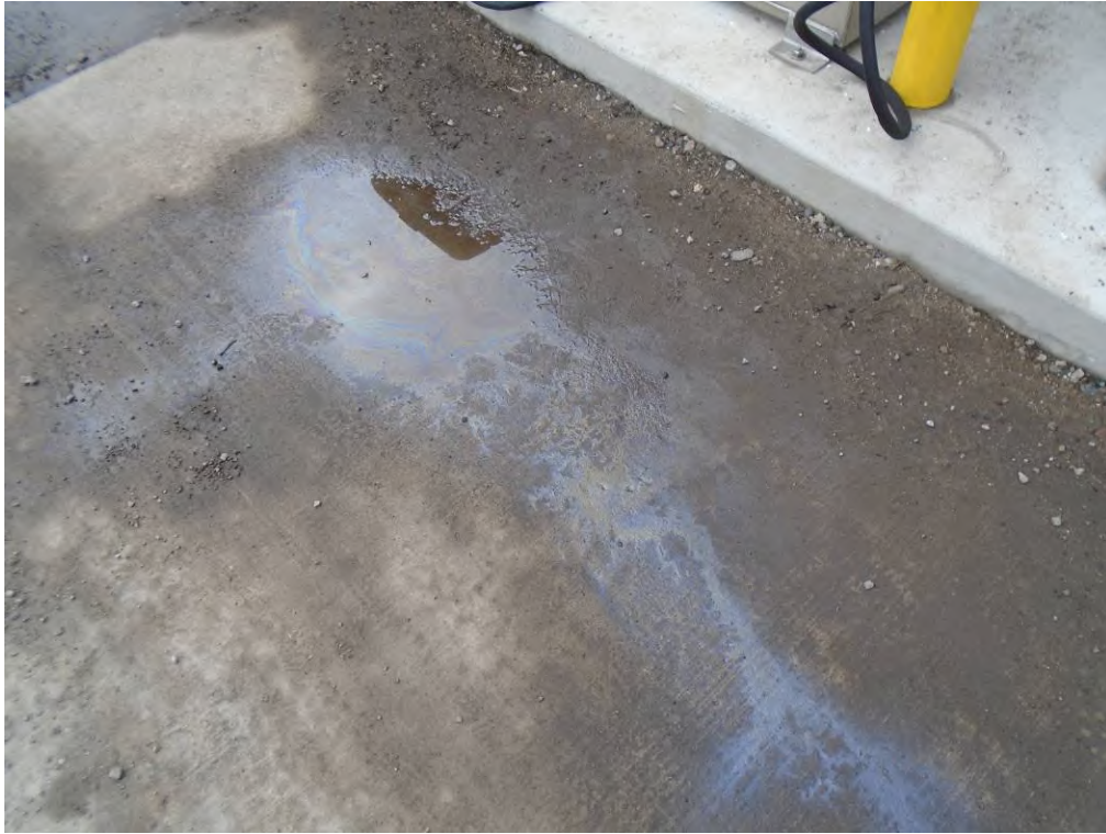
Photo 19: View of surface staining/sheening near the base of the dispenser of the 15,000-gallon diesel fuel AST.
