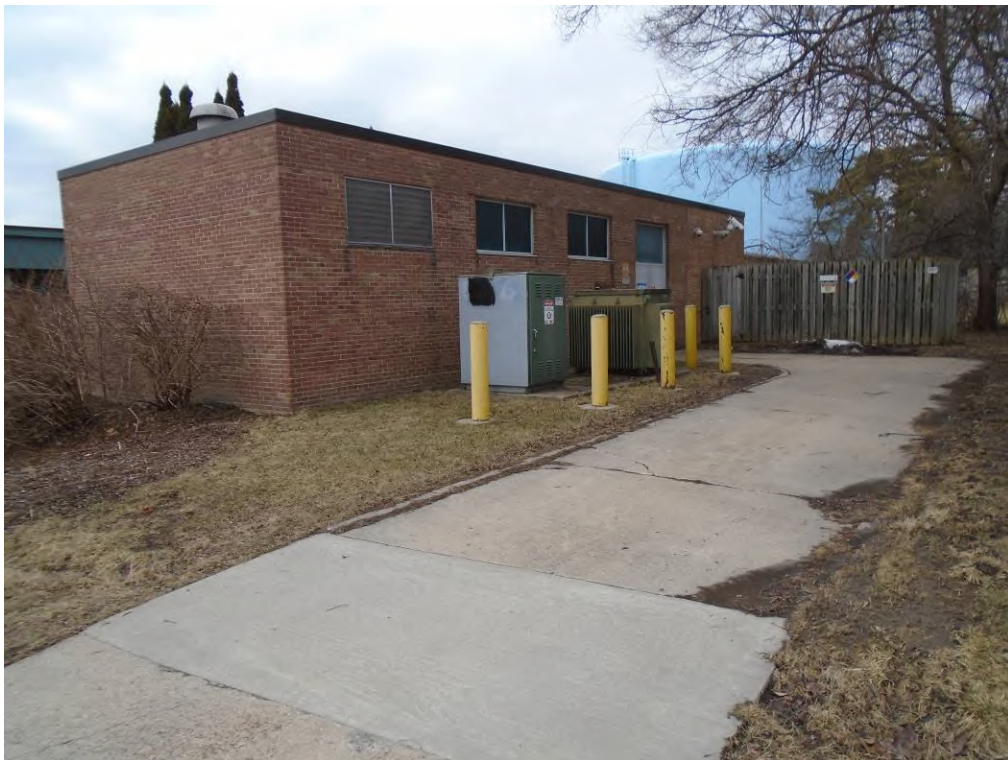
Photo 40: View of northern adjoining property Pump House (1990 S. Industrial).
