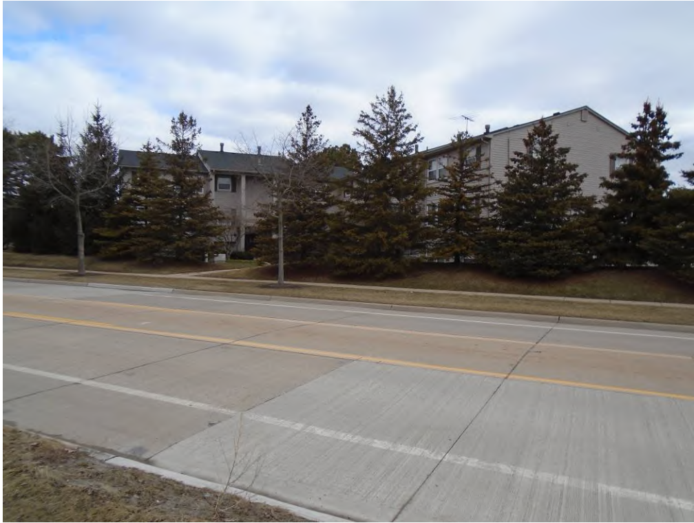
Photo 41: View of northeastern adjacent property Woodbury Gardens Apartments (1208 Astor).
