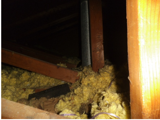
Photo 13: Fiberglass blown insulation in attic
