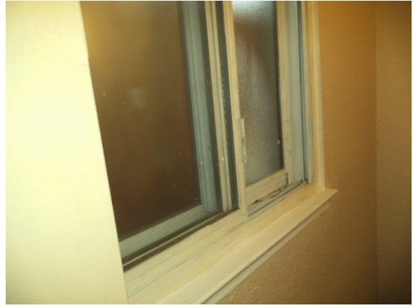
Photo 14: Typical horizontal sliding window frame
