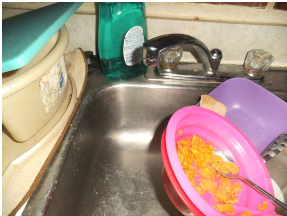
Photo 13: Kitchen faucet and sink
