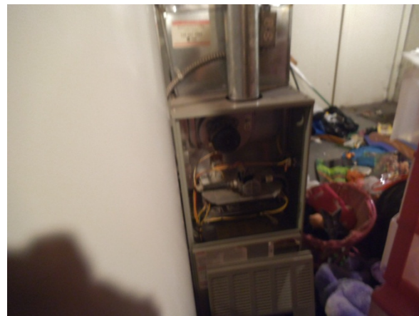
Photo 12: Interior of furnace in basement
