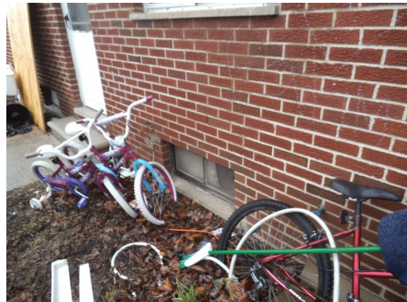
Photo 6: Basement slider windows
