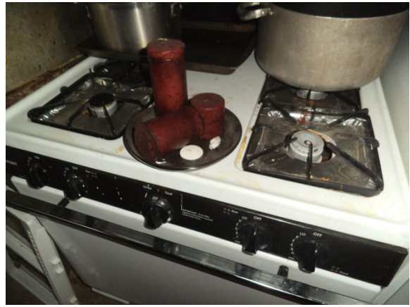
Photo 14: Typical gas stove in unit
