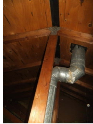
Photo 14: Vent stack to the roof
