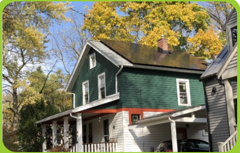
Ann Arbor home generating its own clean energy via solar panels.
