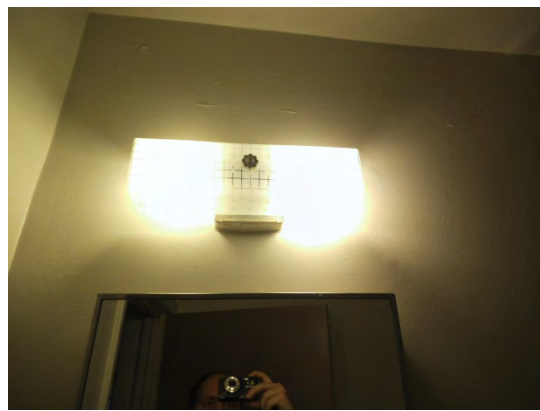
Photo 12: Bathroom light fixture
