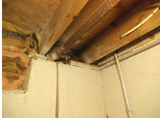
Photo 8: Insulation between basement walls
