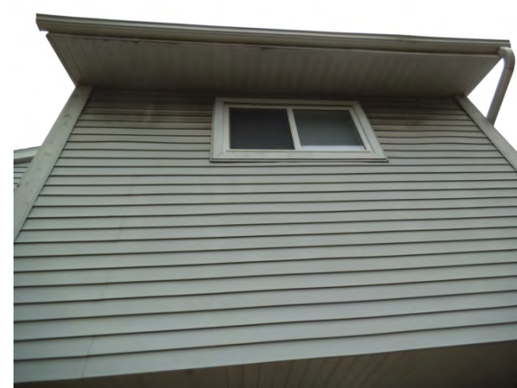
Photo 4: Typical vinyl window
