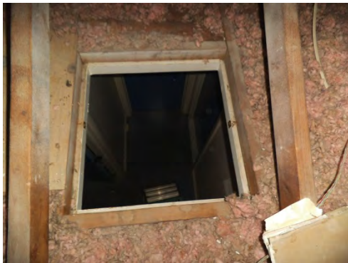
Photo 17: Insulation surrounding attic hatch
