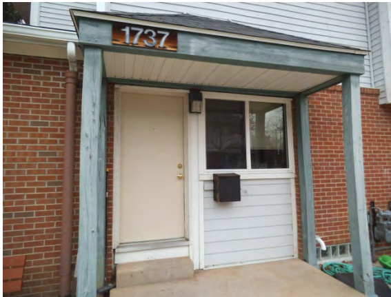
Photo 3: Entrance with exterior lighting
