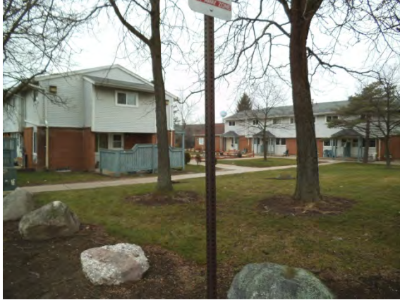
Photo 1: Exterior view of the complex
