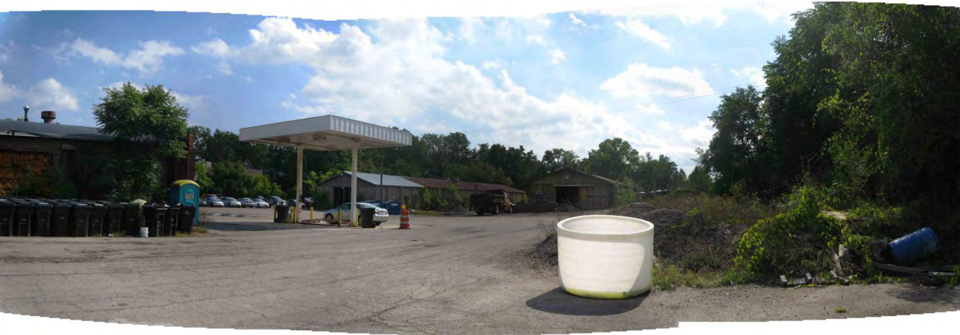
Site interior – from NW corner
