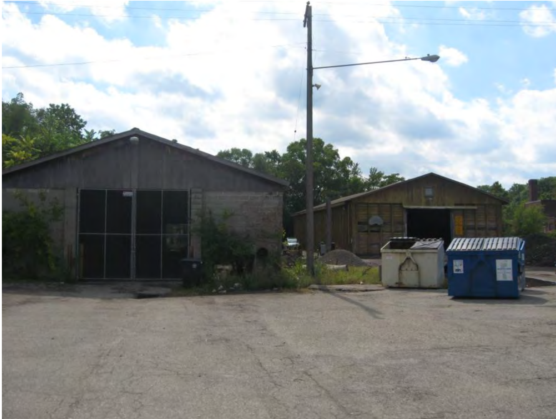
Garage & Salt Storage Buildings (to be removed)
