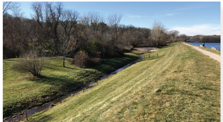
Barton Dam embankment.
