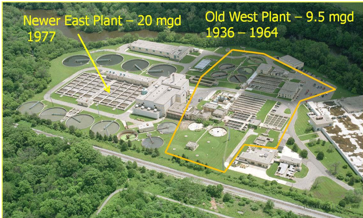
Wastewater Treatment Plant Facilities Renovations Project
