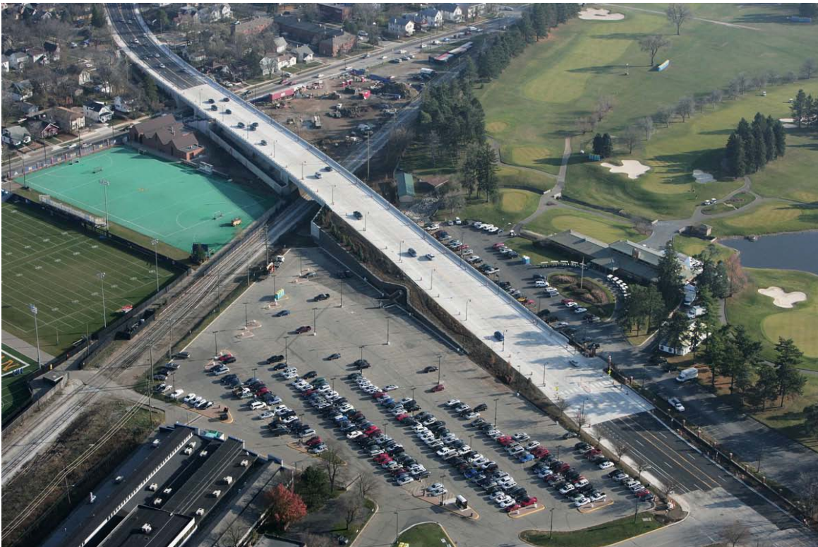
Stadium Bridge Replacement
