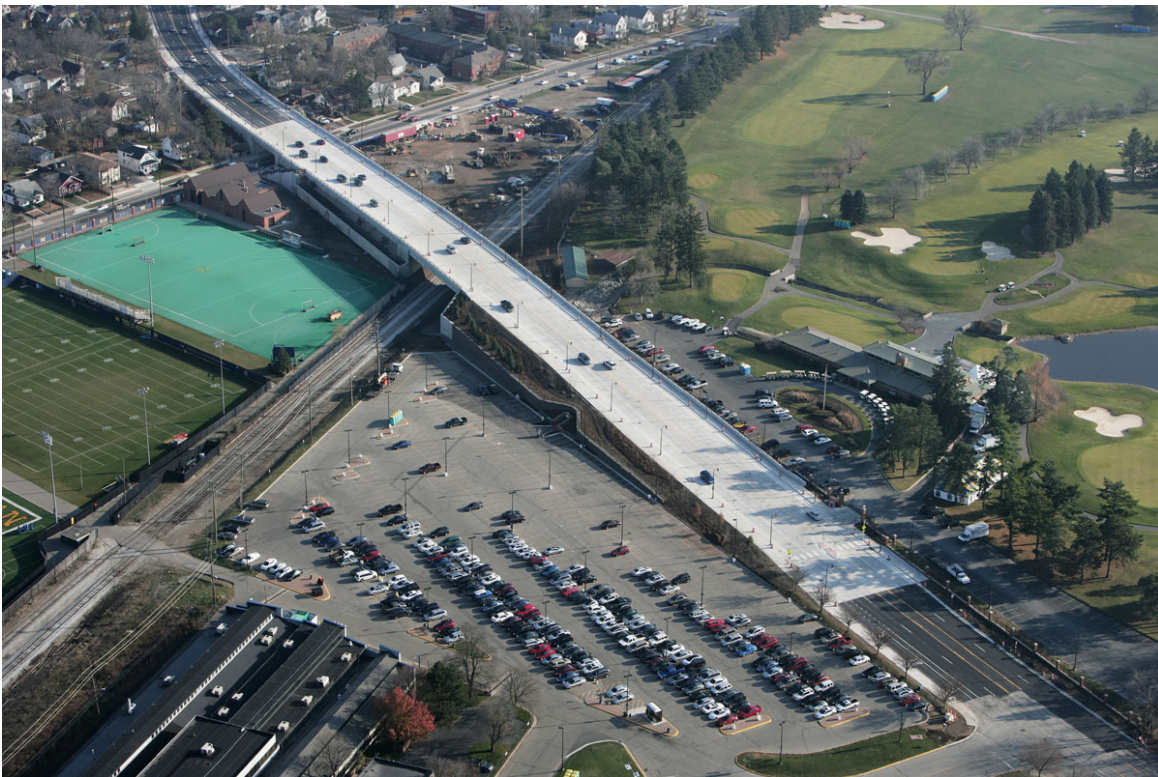
Stadium Bridge Replacement
