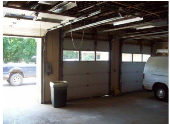
Photo #66: Overhead doors at maintenance shop
