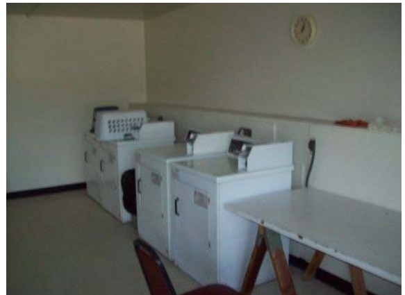
Photo #60: Laundry room dryers
