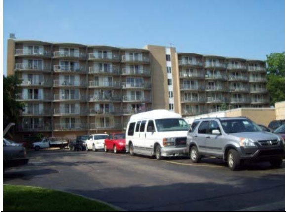
Photo #2: Front elevation of building
