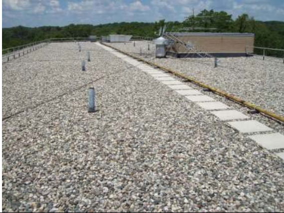
Photo #7: Main roof overview
