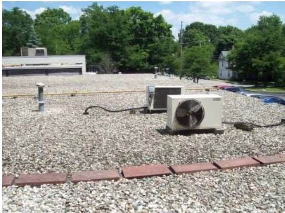
Photo #9: Lower roof detail
