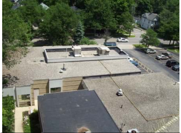
Photo #8: Lower roofs overview
