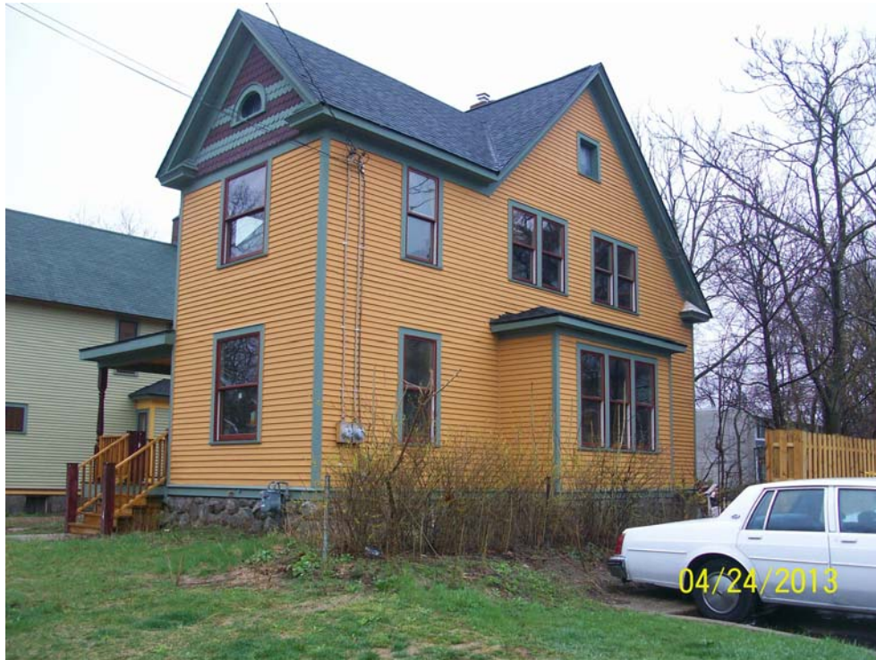
Photograph 31: East adjoining residential house.
