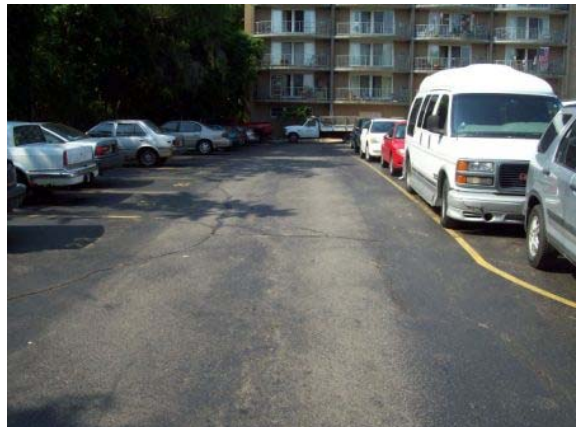
Photo #12: Pavement detail
