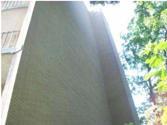
Photo #3: Side elevation of building
