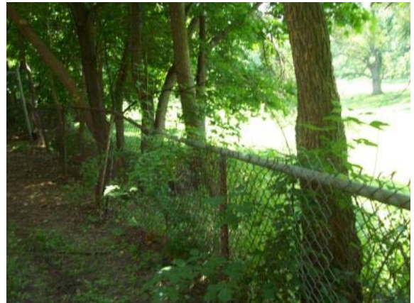
Photo #64: Damaged fencing at south property line
