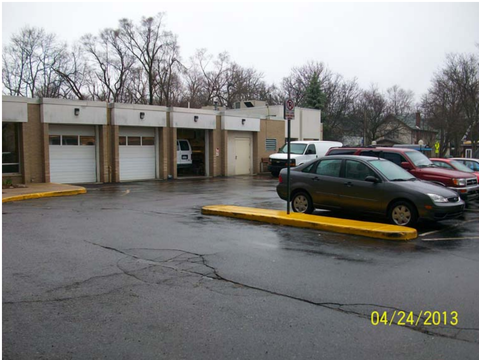
Photograph 26: Garage in the north side addition to the building.
