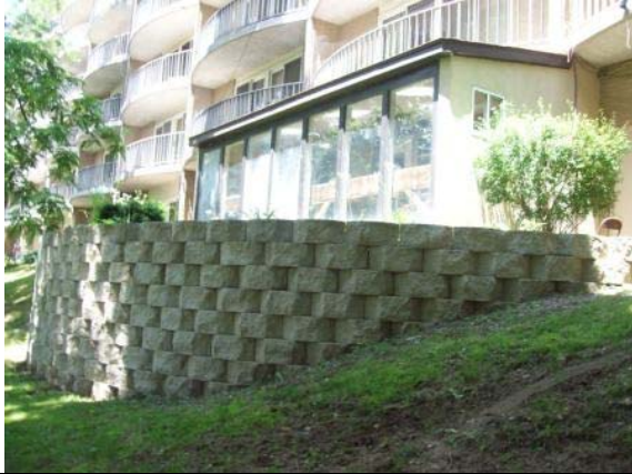
Photo #61: Masonry retaining wall
