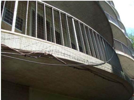
Photo #63: Balcony construction and metal railing
