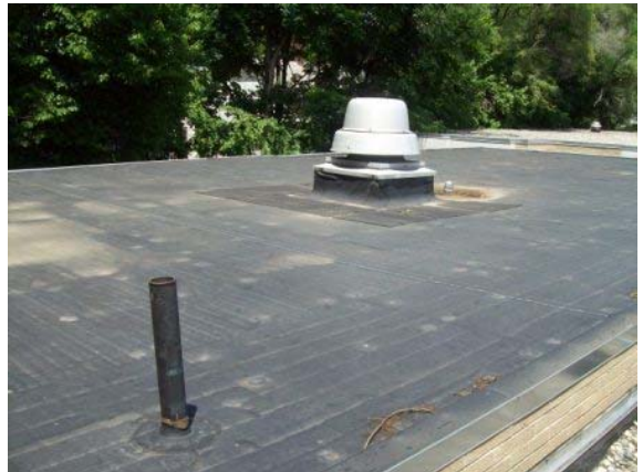
Photo #10: Lower membrane roof detail
