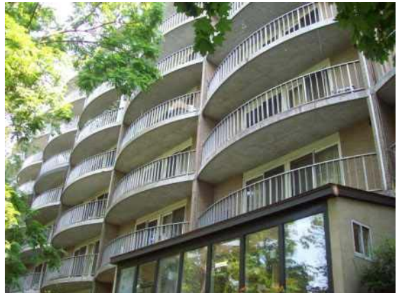
Photo #4: Rear elevation of building
