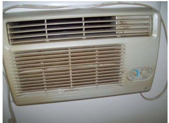
Photo #30: Typical through-the-wall unit air conditioning unit
