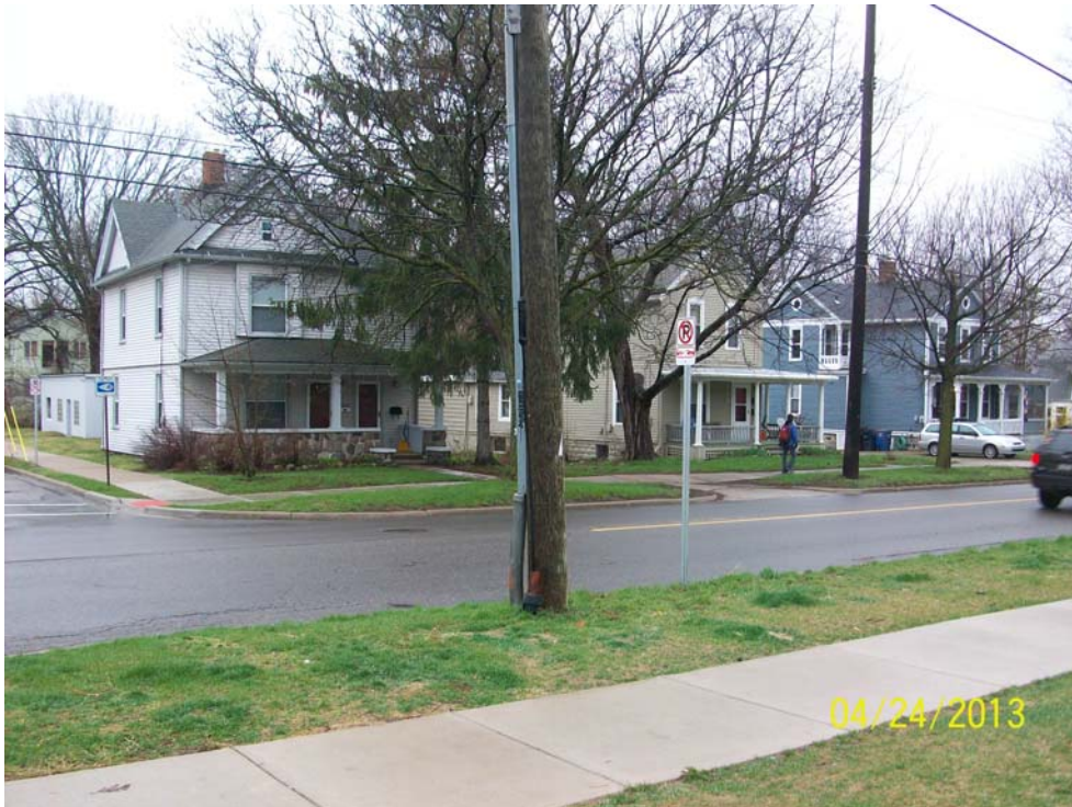
Photograph 28: North adjoining Miller Avenue and residential houses beyond, view facing north northeast.
