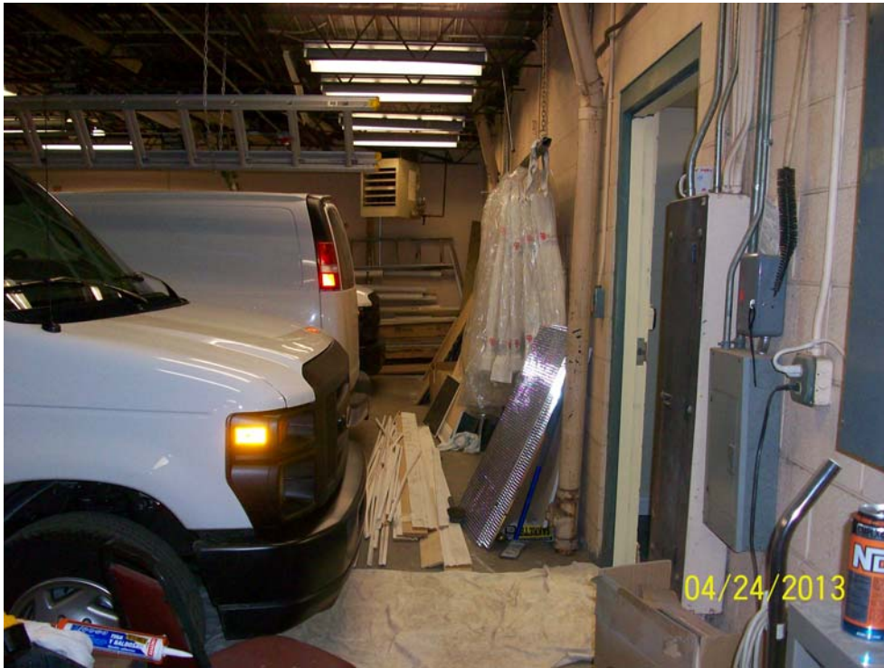
Photograph 25: Vehicle and building component storage in the garage in the north side addition to the building.
