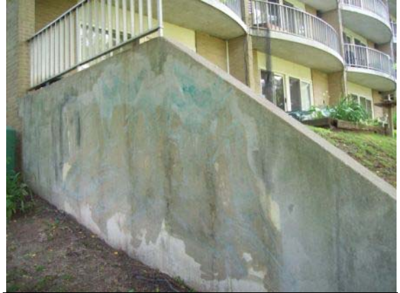
Photo #62: Concrete retaining wall
