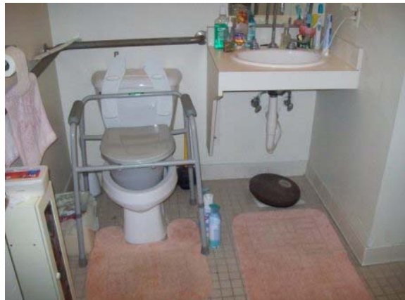
Photo #24: Accessible unit bathroom
