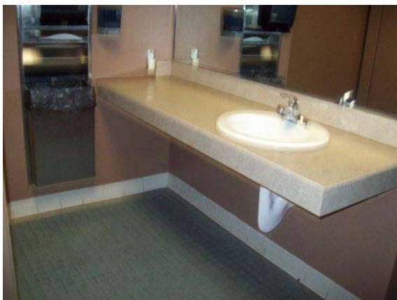
Photo #17: Common area restroom
