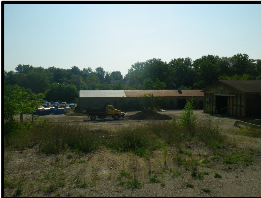
Looking east at the garbage barn and wooden barn
