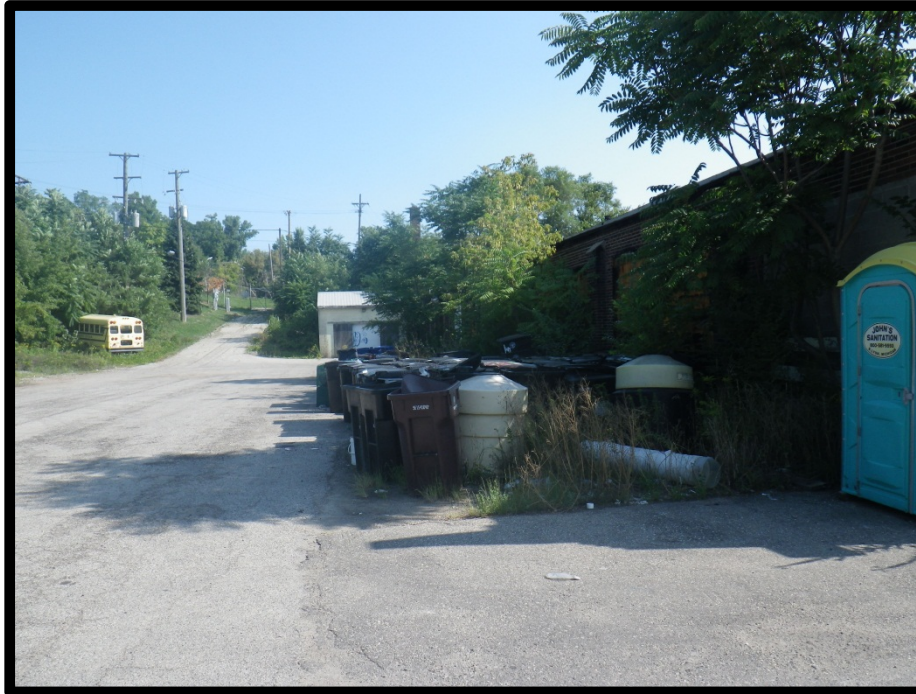
Looking north, along the west side of the maintenance building and former location of 16,000 gallon AST
