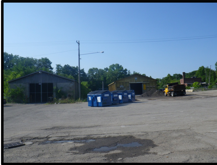
Looking south at the garbage barn (left) and the wooden barn (right)
