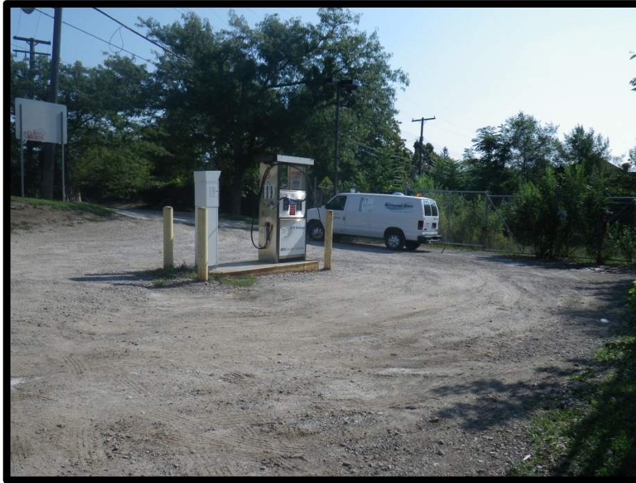
Compressed natural gas station located along Summit St.
