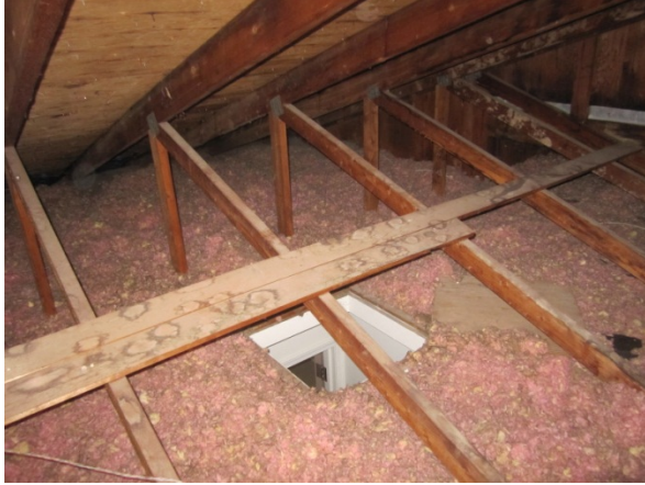
Photo 19: Insulation near attic hatch
