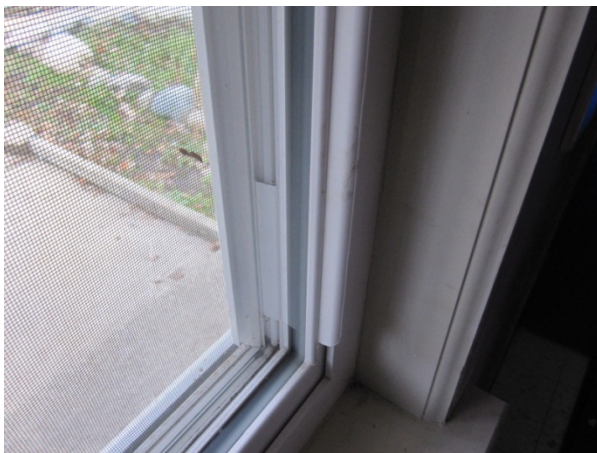
Photo 11: Vinyl windows in Community Center
