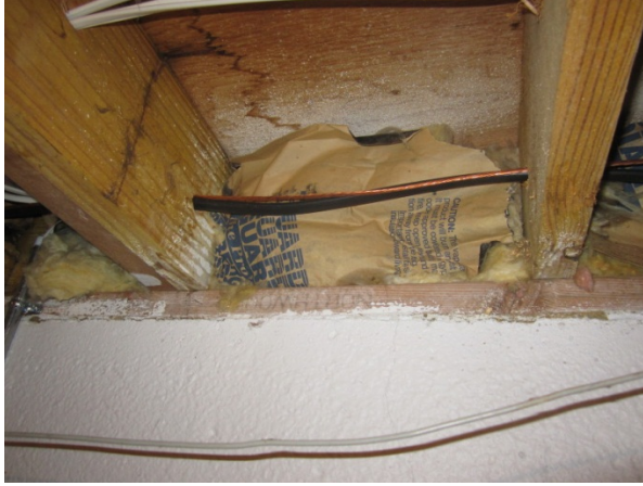
Photo 13: Insulation in between floor joists in basement
