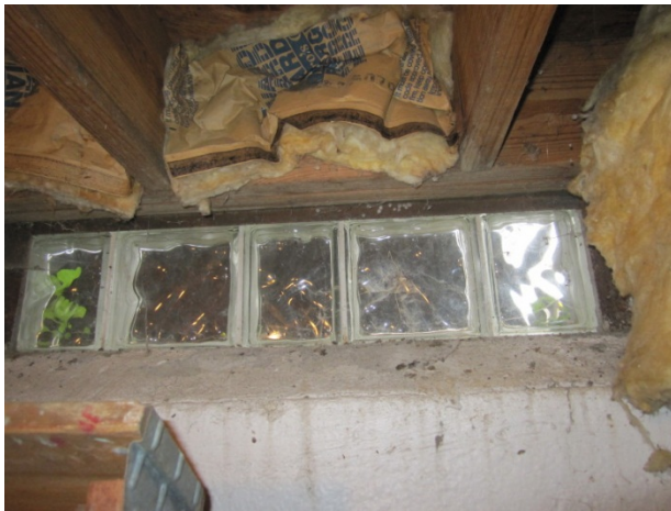
Photo 15: Basement glass block windows
