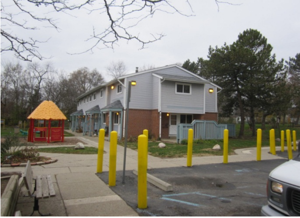
Photo 1: Exterior view of complex from parking lot
