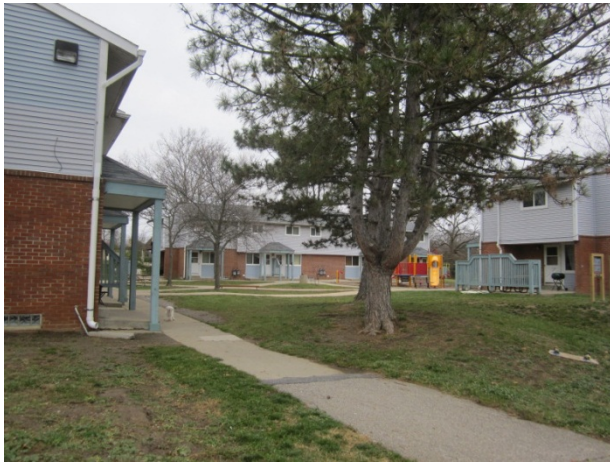
Photo 3: Exterior view of complex
