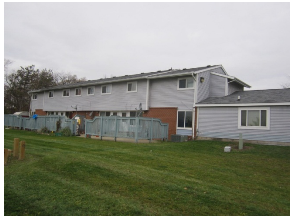
Photo 2: Exterior back side view of complex
