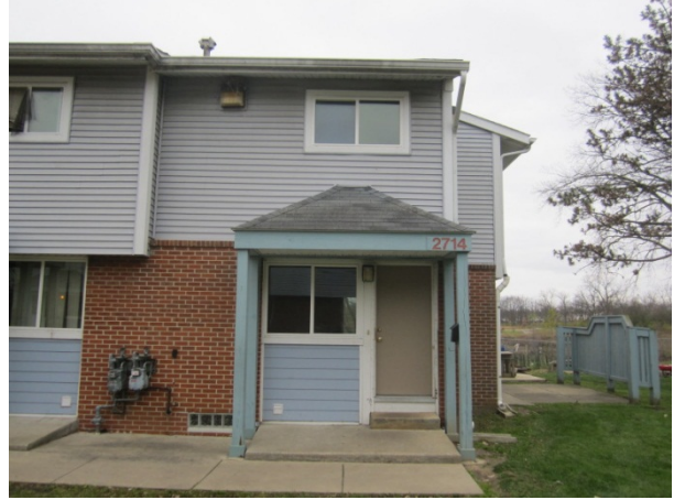
Photo 20: Sample unit used for blower-door test
