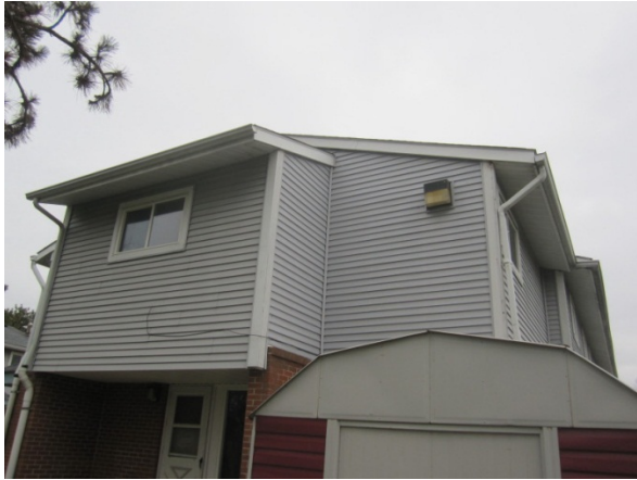
Photo 21: Exterior wall-mounted lighting
