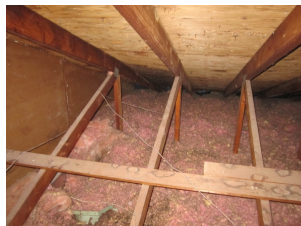
Photo 18: Insulation in attic space
