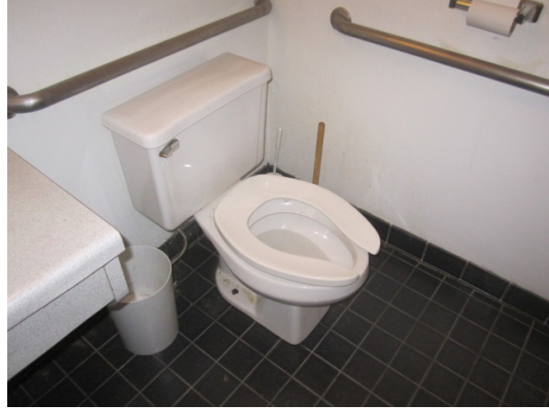
Photo 8: Typical Bathroom Toilet
