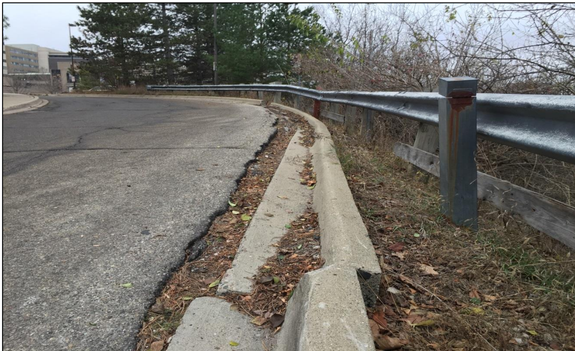
PHOTO NO. 8: Looking west along the north curb line of Nichols Drive. Inclinometer I-2 is in the right of the photo between the curb line and the guardrail.
