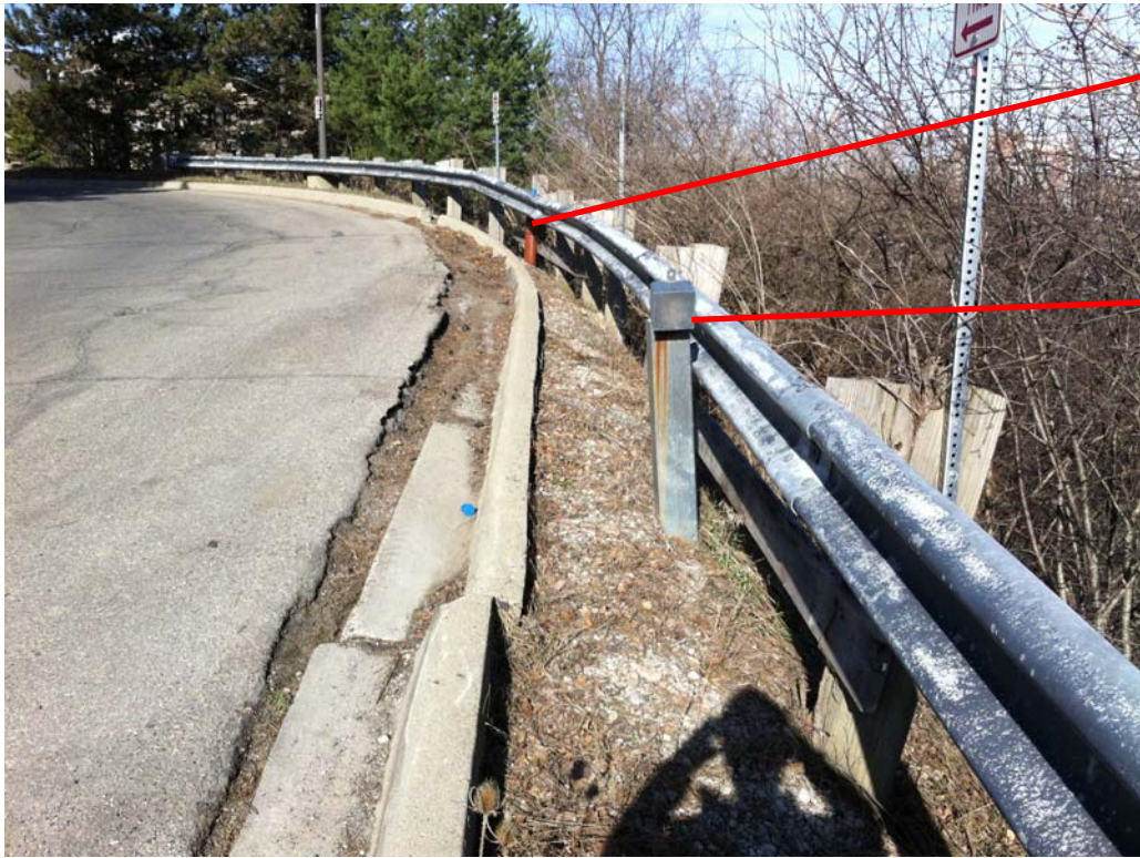
2014 Looking west, toward inclinometers I-1 and I-2 [provided for comparison]
