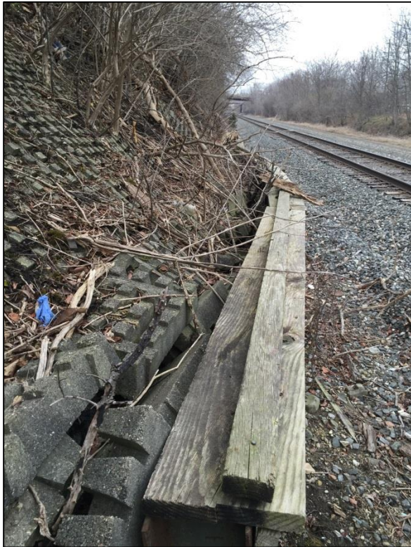
PHOTO NO. 10: Looking west along the top of the soldier pile retaining wall at the toe of the slope.
