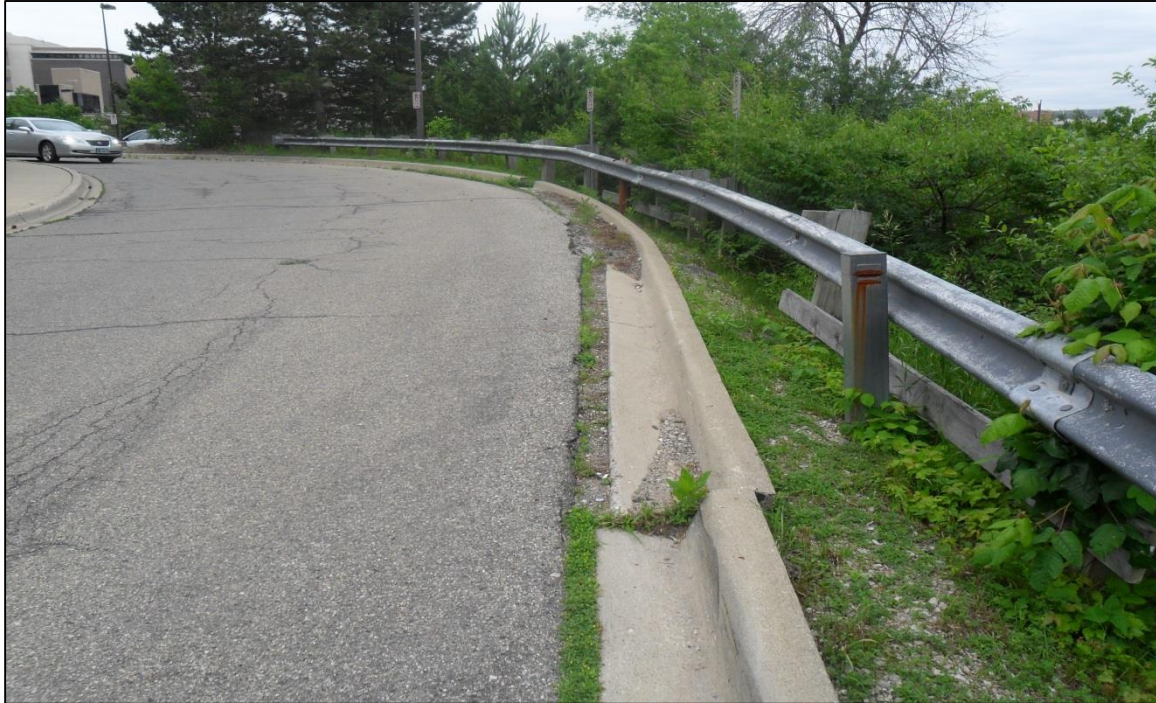
PHOTO NO. 1A – June 11, 2010: Looking west along the north curb line of Nichols Drive. Inclinometer I-2 is in the right of the photo between the curb and the guardrail.
